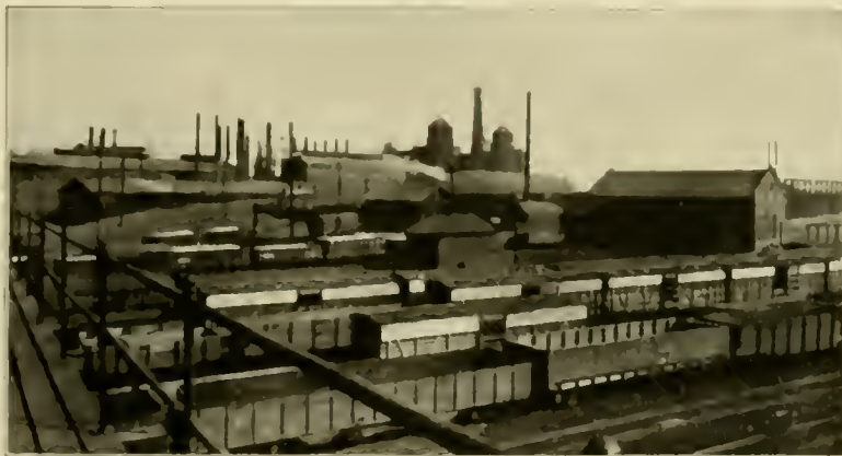
FIG. 38. A general view of the Illinois Steel Works at South Chicago.
