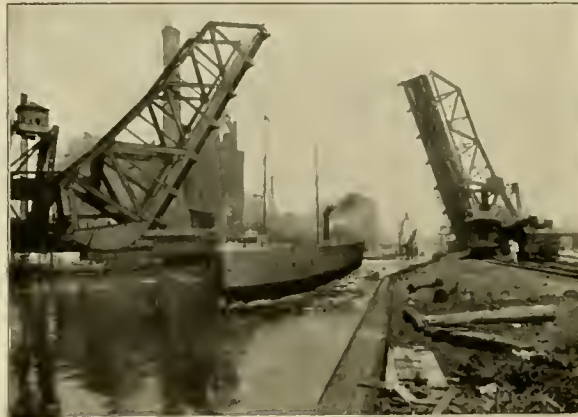
FIG. 35. Through the manufacturing district of Chicago. The picture shows the bascule bridge at 12th Street open to allow a lake steamer to pass.
