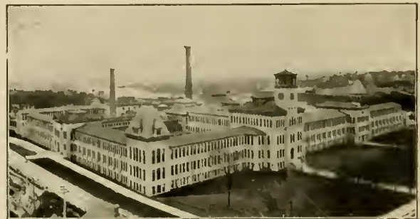
FIG. 36. The plant of the Elgin National Watch Company, Elgin, Ill.
