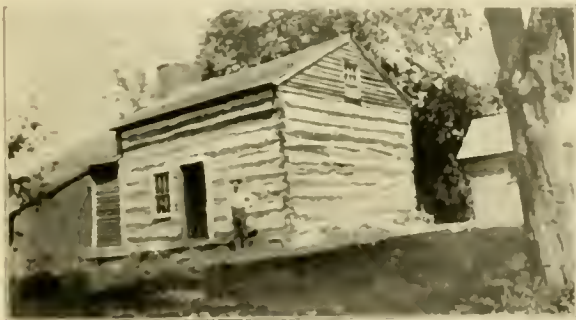
FIG. 17. A typical early settler's cabin in Illinois. Notice the logs chinked with plaster, and the old stone chimney. The outbuildings are modern.
