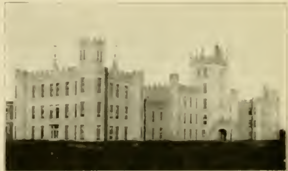
FIG. 56. The Northern Illinois State Normal School at Decatur.
