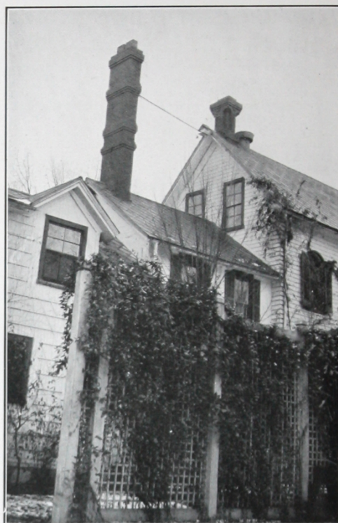
FIG. 10. SHOWING EXTENSIONS TO THE CHIMNEY REQUIRED IN ORDER THAT IT MIGHT DRAW PROPERLY.
