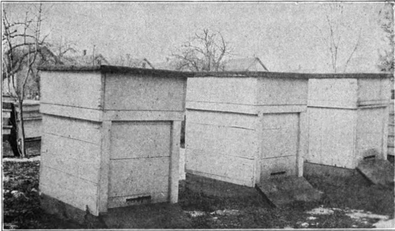
Fig. 132—G. C. Greiner's Double-Walled Hives Made of Dry-Goods Boxes.
