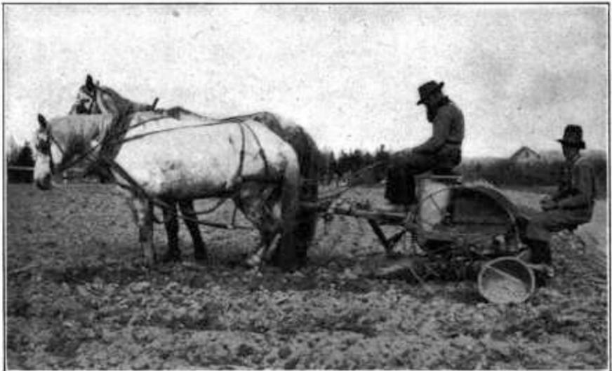
FIG. 3.—Potato planter of the type operated by two men.
