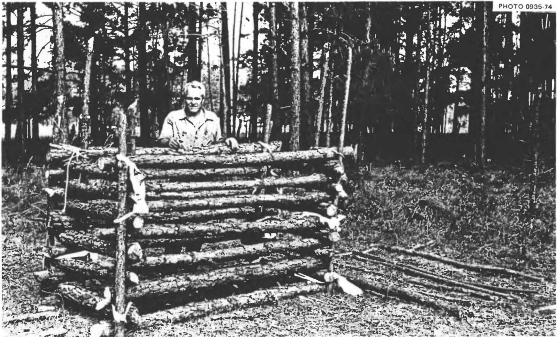
5.26. A different crib design that requires no notching of poles. Note the two vertical, small-diameter poles tied into each corner, one inside the crib, and the other outside. Each pair of vertical small poles was tied together (top, center, and bottom) with three "ropes" made of foot-wide strips of bed sheet, or (at only two points) with rope.
