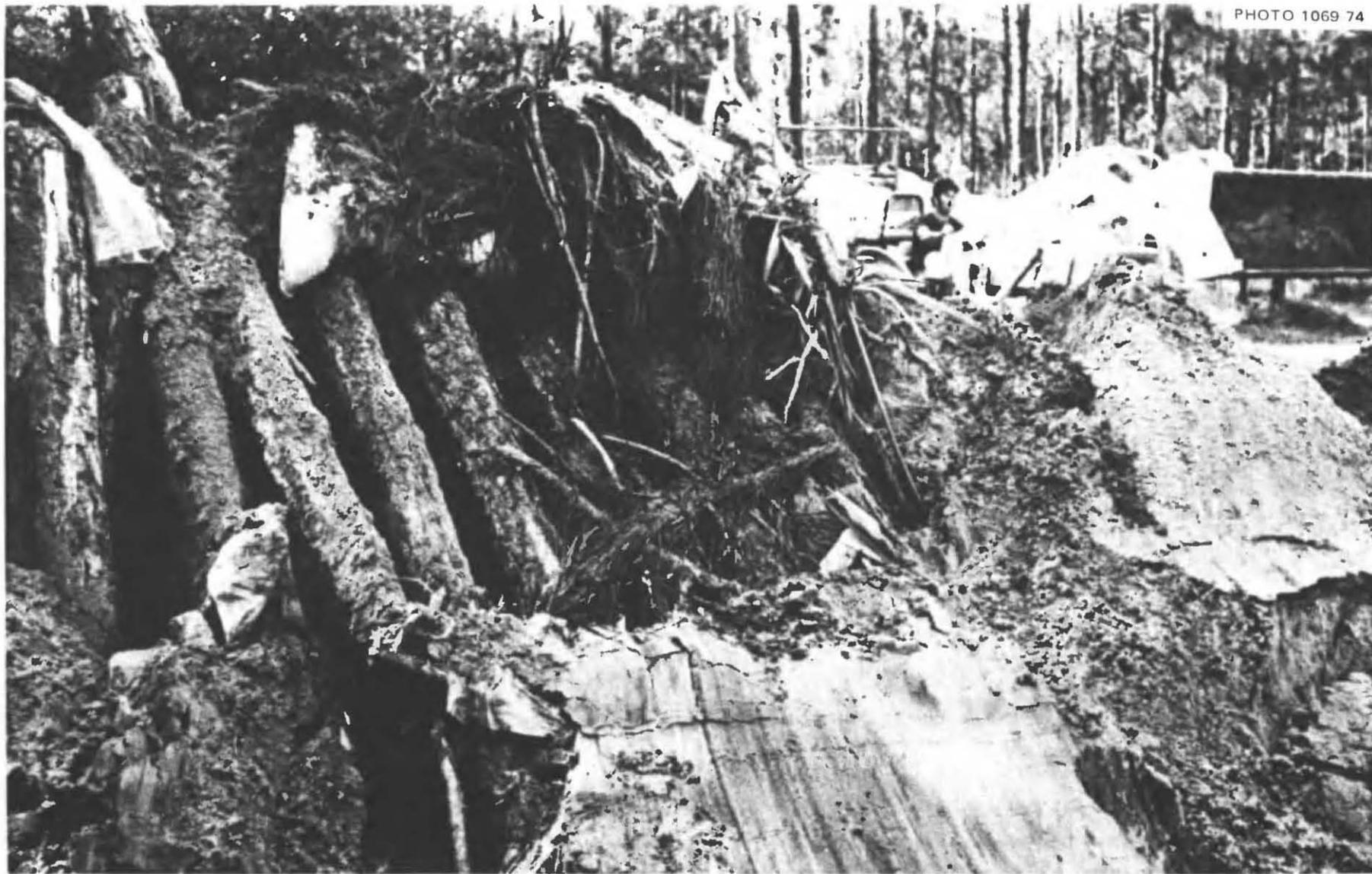
**Fig. 5.40.** View after a backhoe had started to demolish the Waldens' Ridge-Pole Shelter, which proved to be decidedly sturdy. Note that some of the wall poles were broken before they were moved off the ridge poles, or the ridge pole had been moved significantly.
