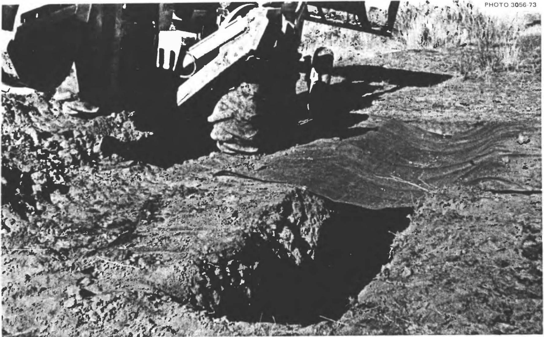
Fig. 3.12. Compacting the earth over one edge of the tarp. This edge has been placed in one of the two 16-in.-wide by 12-in.-deep rectangular trenches, each of which was dug parallel to and 3 ft from the vertical walls of the shelter trench. Packing with this wide-wheeled backhoe did not compact the earth as well as hand-tamping it with a pole.
