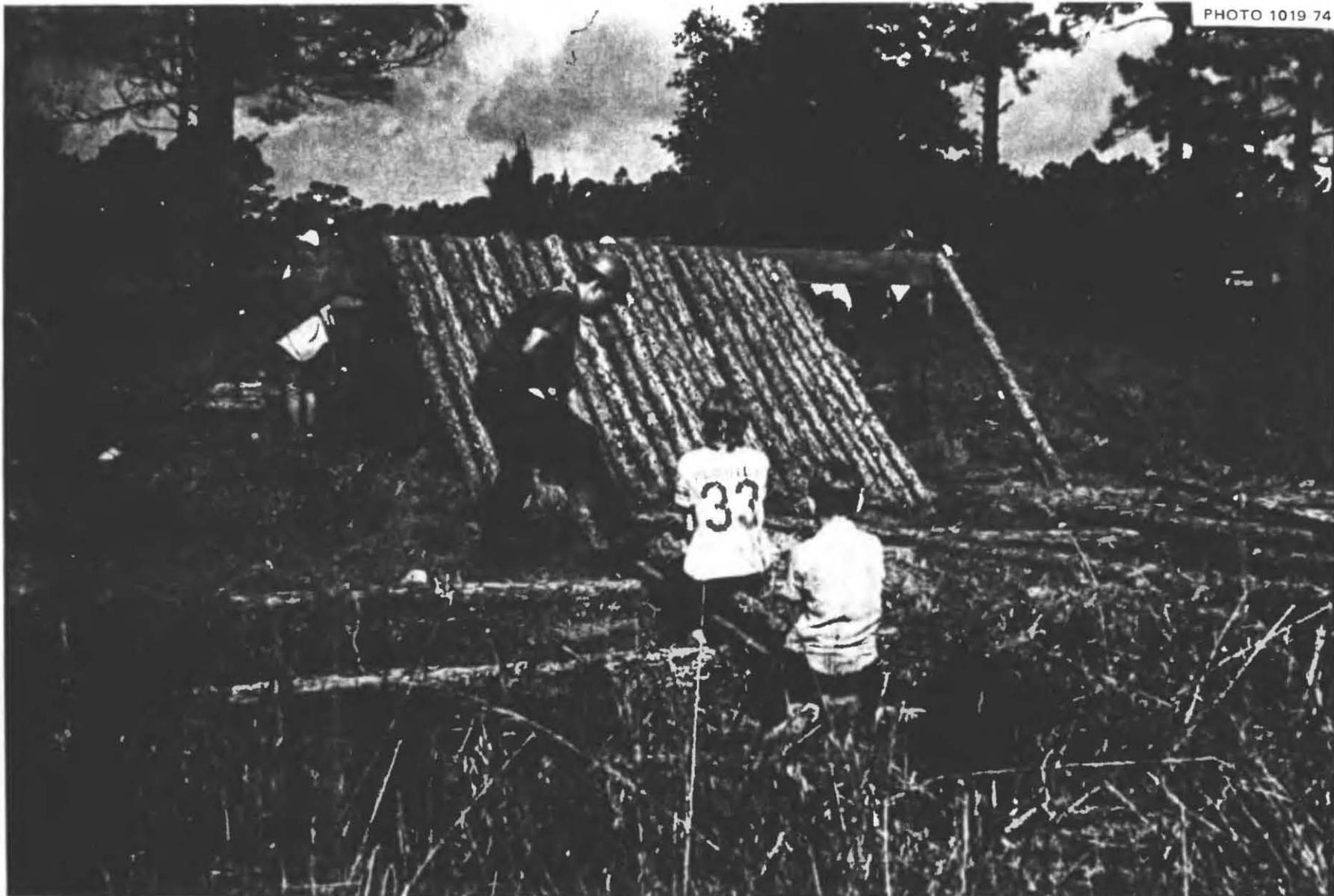
Fig. 5.45. Chain saw operator using a templet to cut an upper end of a wall pole at the specified  $54^\circ$  angle and 9-ft length on its short side. The templet was made from a wide 10-ft board, with one end cut at  $54^\circ$ . A nail was driven 9 ft from the end of this  $54^\circ$  angle; the squared-off base of the pole was placed against this nail.
