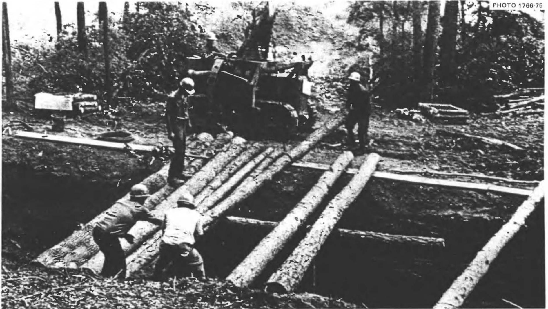
Fig. 7.1. Workmen of a pipeline contractor laying 22-ft logs across a 12-ft-wide bulldozed trench. This trench was bulldozed 7 to 8 ft deep into firm, weathered-in-place Alabama clay. The sides of the trench were vertical.
