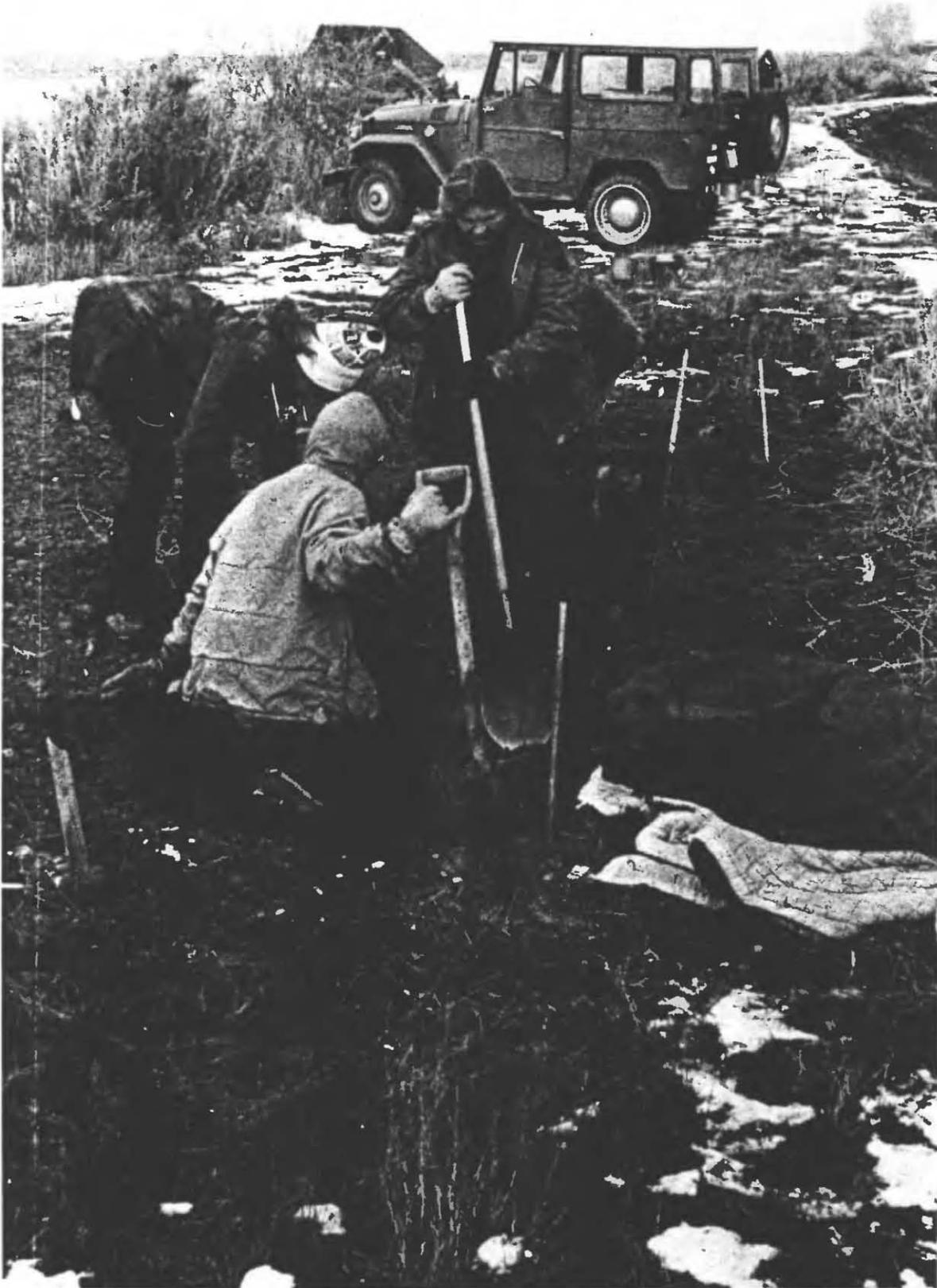
Fig. 2.5. Instead of sharpening their pick and using it, this family mostly pried and scraped away the dry, hard clay-loam with shovels, inch by inch.
