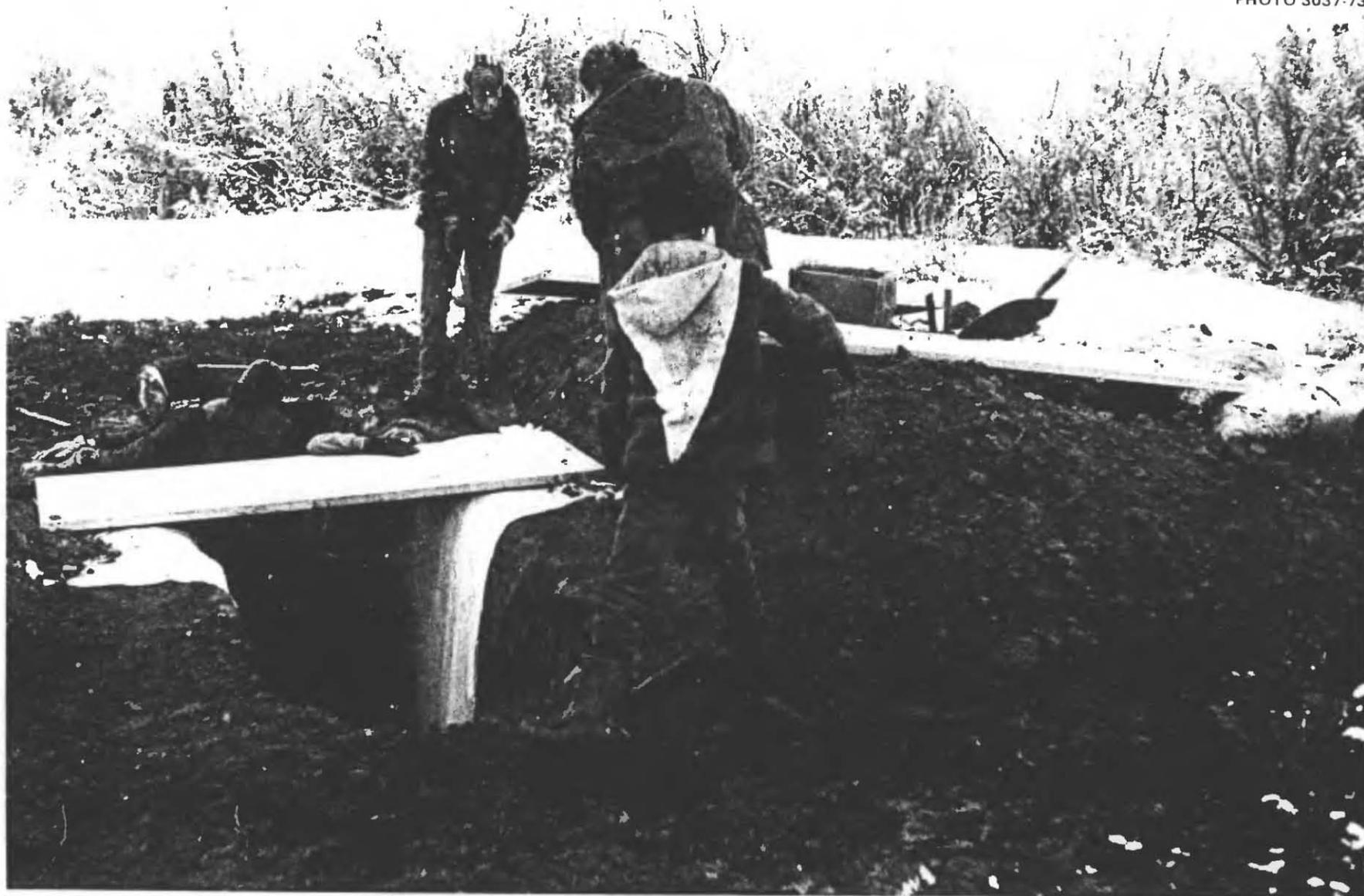
Fig. 2.9. Placing the first of six interior, hollow-core doors over the completed trench. The earth on the wall-lining sheet was removed before the second door was positioned.
