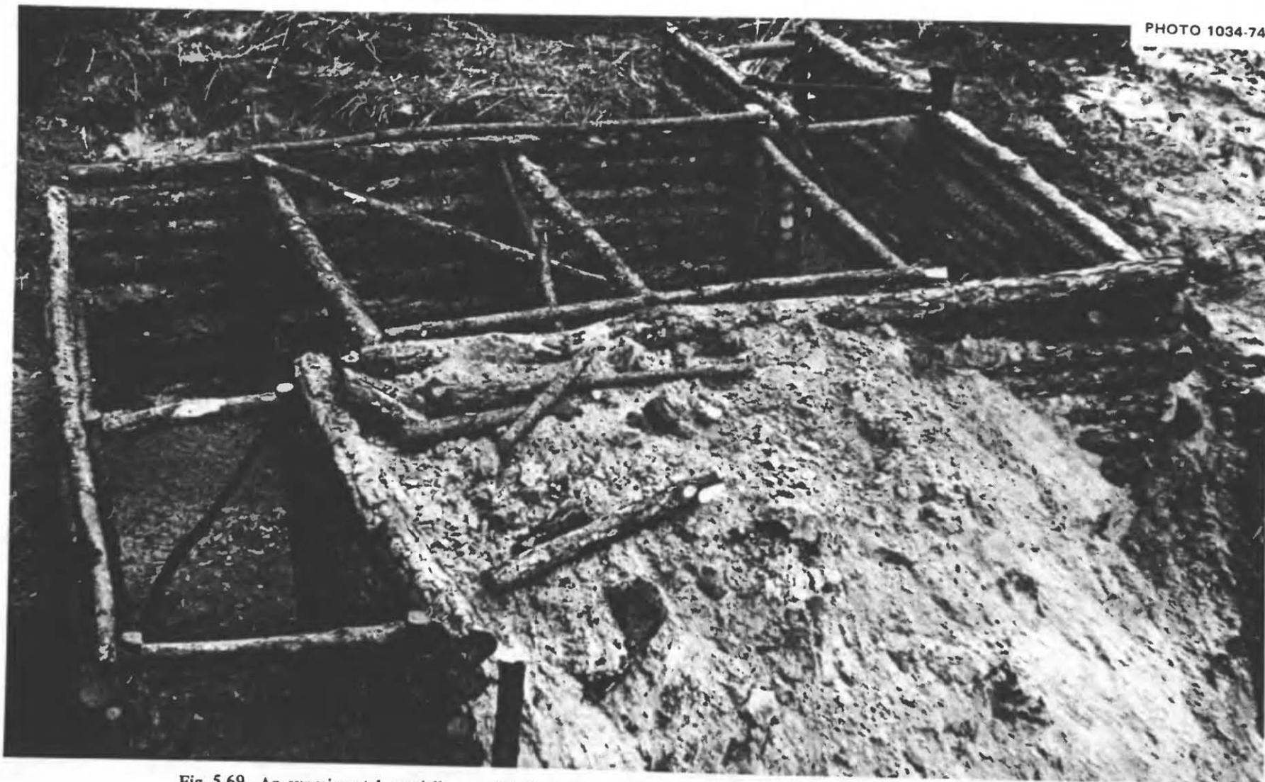
**Fig. 5.69.** An experimental, partially completed, prototype stoop-in pole shelter designed by Kearny with horizontal wall poles, in order to minimize the cutting of poles needed to build a given area of walls. After the level of the earth mounded around this shelter had been raised about 3 in. higher than the uppermost poles, the 6-ft-wide shelter was roofed with 9-ft poles resting on the mounded earth. Then 2 ft of earth cover was placed on the roof.
