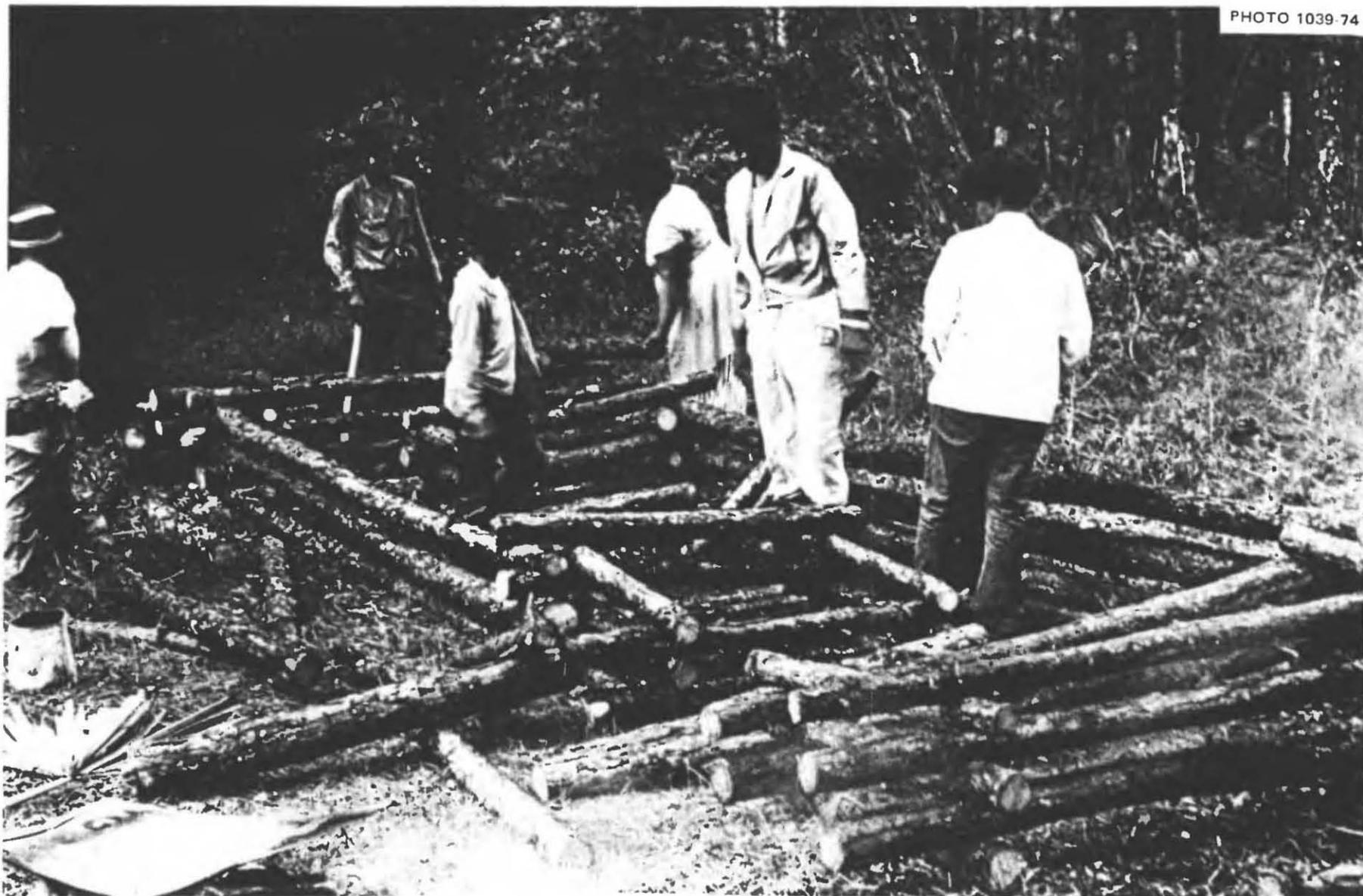
**Fig. 5.16. Building the cribs forming the entrances and ends of this shelter, and also making the connecting spaced-pole walls of the main room.** This family of 6 consisted of a father, aged 55, who is a painter and odd-job handyman; a mother, aged 50, who is a school custodian; a son and daughter, both 16; and two small but strong sons, aged 13 and 11.
