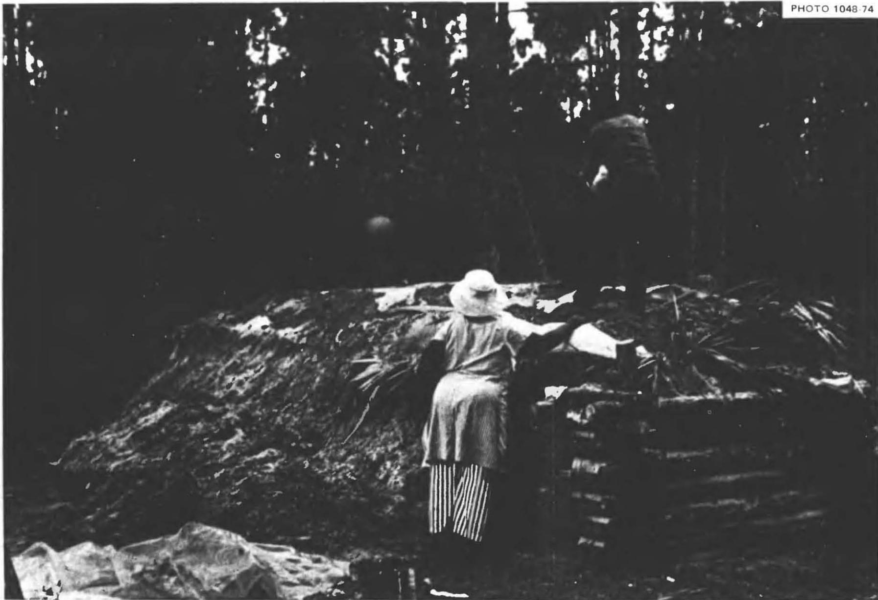
Fig. 5.23. After mounding earth over the shelter roof so that the earth was about 1 ft deep over its centerline, this family made a rainproof "buried roof" out of waterproof material. Since they had part of the north side of their home covered with a big piece of polyethylene film to keep the winter wind from blowing through cracks, they had enough waterproof material to bring with them to the shelter-building site to cover this entire shelter roof.
