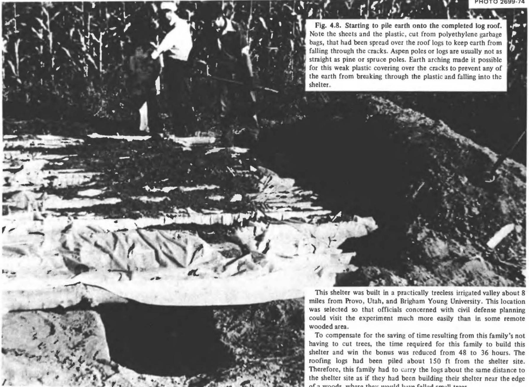
Fig. 4.8. Starting to pile earth onto the completed log roof. Note the sheets and the plastic, cut from polyethylene garbage bags, that had been spread over the roof logs to keep earth from falling through the cracks. Aspen poles or logs are usually not as straight as pine or spruce poles. Earth arching made it possible for this weak plastic covering over the cracks to prevent any of the earth from breaking through the plastic and falling into the shelter.
