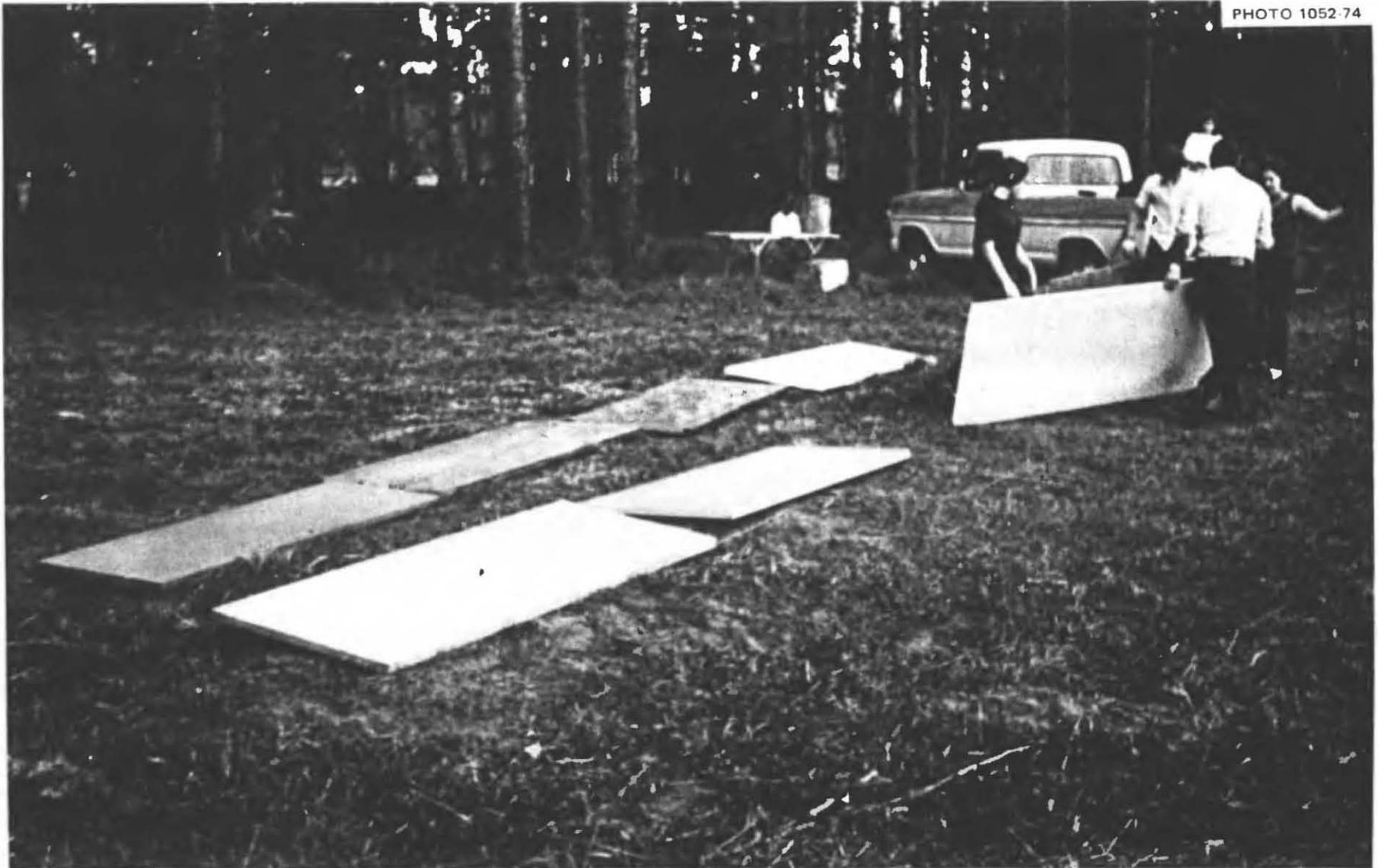
**Fig. 5.2.** The start of an expedient-shelter-building test by a family from Bunnell, Flagler County. In this test an inexperienced family, guided only by illustrated written instructions, built an above-ground shelter using interior hollow-core doors for the roofing material. The walls were made of earth-filled rolls made of bed sheets, as detailed in the drawing for this shelter. Only materials found in most urban homes were used.
