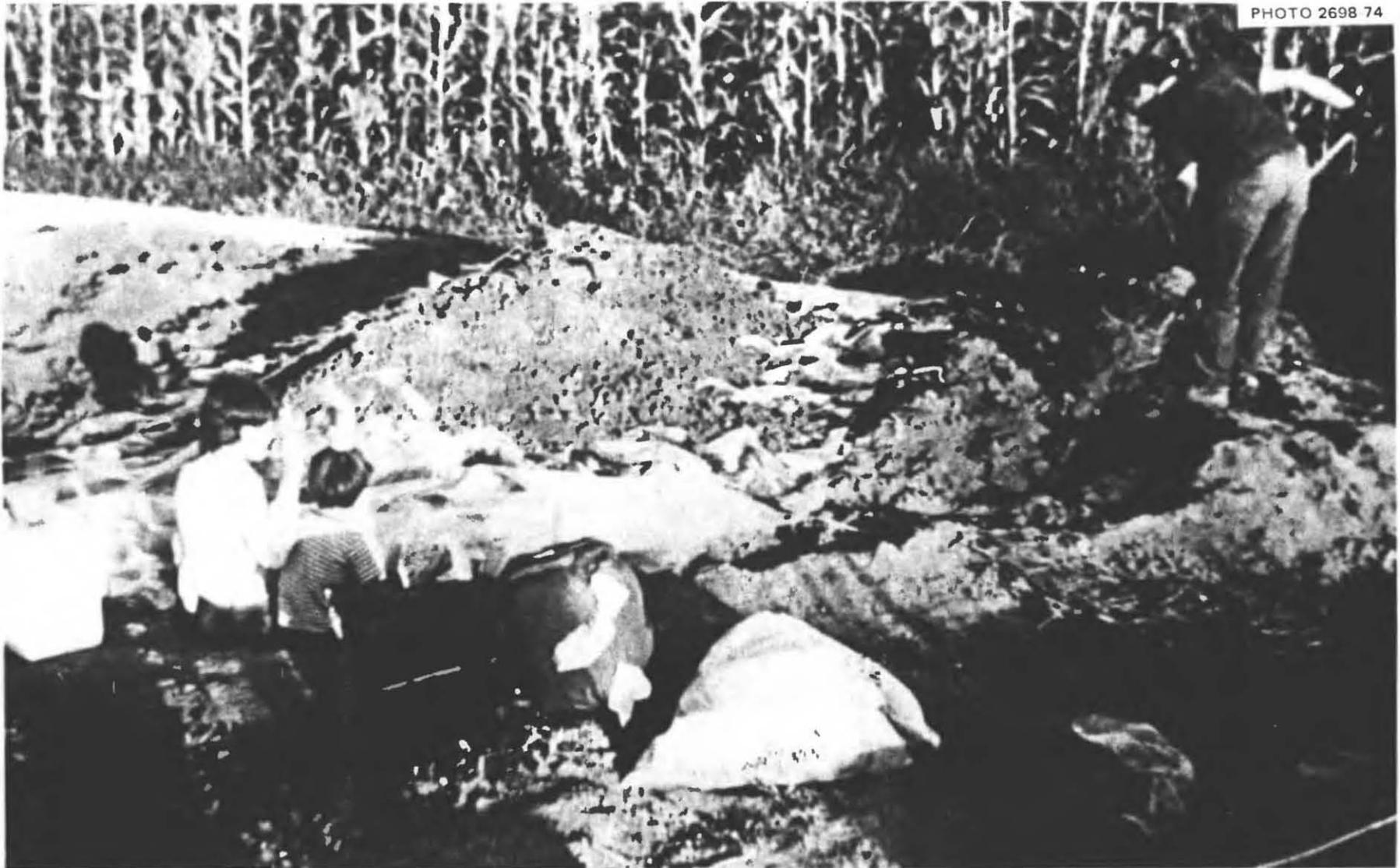
Fig. 4.9. Shoveling earth onto the "buried roof" made of a large piece of 4-mil polyethylene. After earth had been mounded onto the roof logs until it was about 18 in. deep along the centerline, the polyethylene sheet was spread over the entire roof area.
