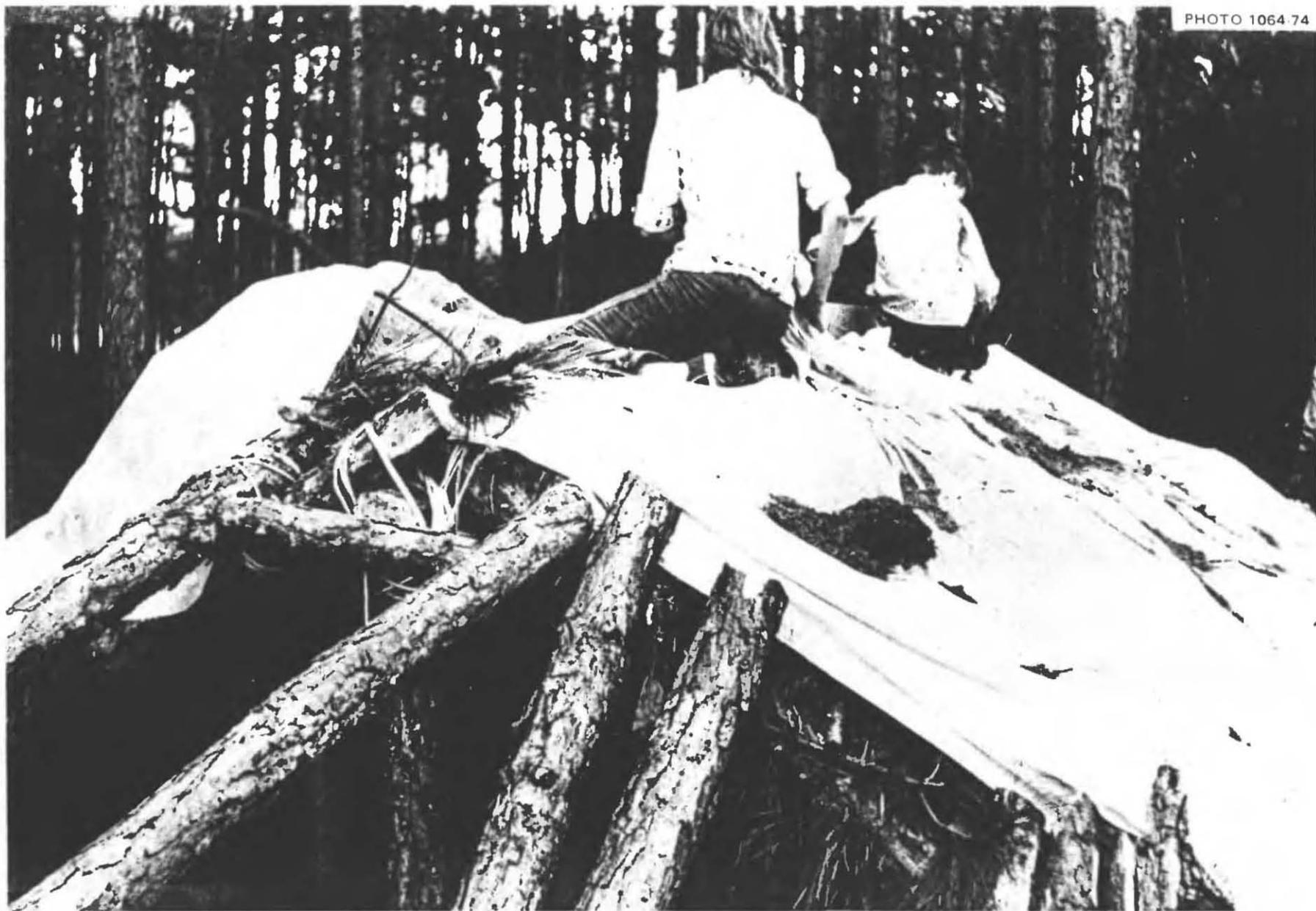
Fig. 5.34. Placing bed sheets over the pine limbs that had been placed crosswise over the roofing poles of the shelter. After the whole shelter had been covered in similar fashion, earth was shoveled or carried so as to cover the entire shelter. This covering was done from ground level upward.
