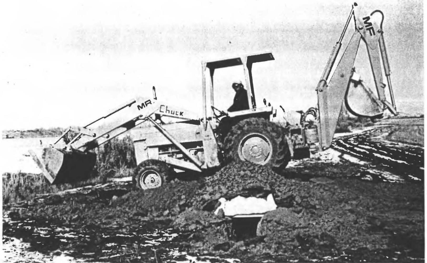
Fig. 3.5. In order to break the roofing doors, the backhoe removed all but about a 2-ft thickness of the earth covering. Then the 8-ton backhoe was driven over the shelter; this compacted the earth under the wheels (reducing its thickness to  $21\frac{1}{2}$  in.) and suddenly broke the  $\frac{1}{8}$ -inch mahogany veneer on the lower sides of two doors. But the  $\frac{1}{8}$ -in. veneer on the upper sides of the doors did *not* break!
