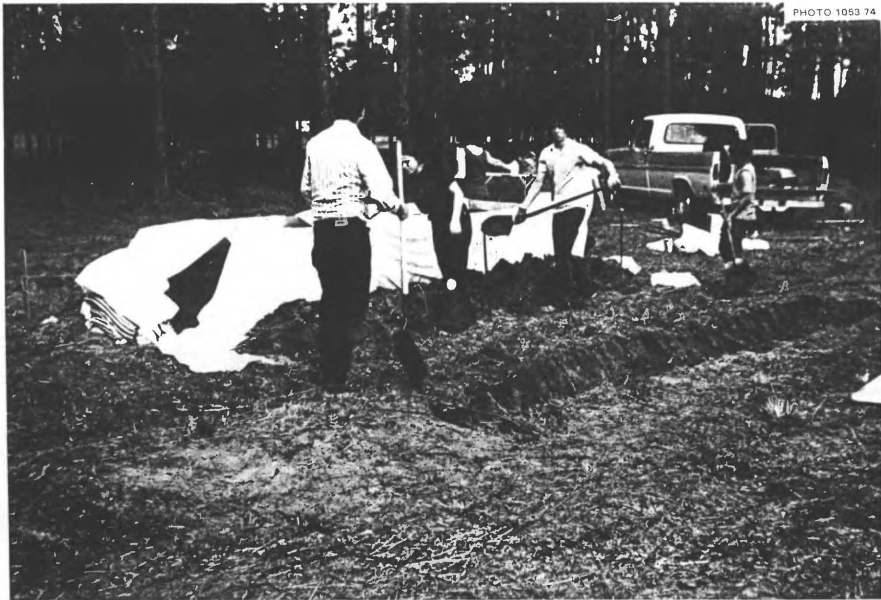
Fig. 5.4. Starting to make the first roll by shoveling earth onto bed sheets that had been placed with 2 ft of their long sides on the ground, with the rest of the sheets temporarily draped over the doors used as forms. This sandy earth could be dug quite easily with shovels.
