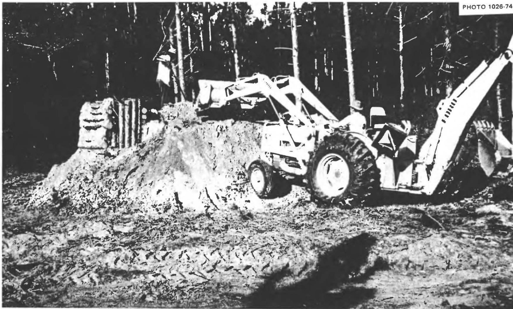
**Fig. 5.68.** Backhoe covering the unsuccessfully modified Small-Pole Shelter with three rooms built entirely above ground. The backhoe worked for almost 5 hours to place earth on this shelter to a minimum depth of 2 ft, because it could excavate only a little over a foot deep without getting stuck. The backhoe repeatedly had to lift itself out of the mud on both its buckets, although this work was done toward the end of a long dry spell.
