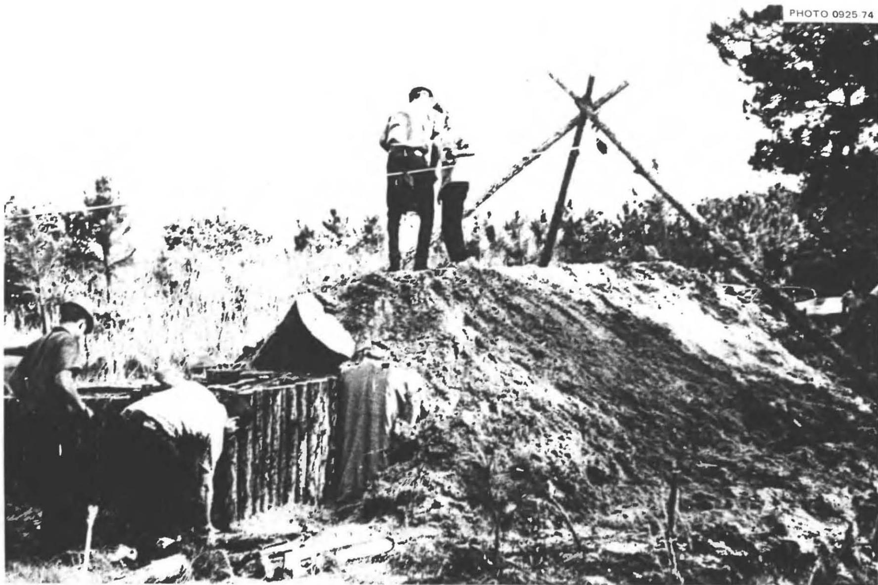
Fig. 5.51. The pulley conveyor system actually wasted energy and time, since earth had to be lifted in a 5-gallon paint can up to the hook on the movable pulley; then the earth-filled can was pushed up the upward-sloping nylon rope to a position several feet above the top of the shelter. Then most of the earth rolled down below the top of the shelter, obviously wasting thousands of foot-pounds of work.
