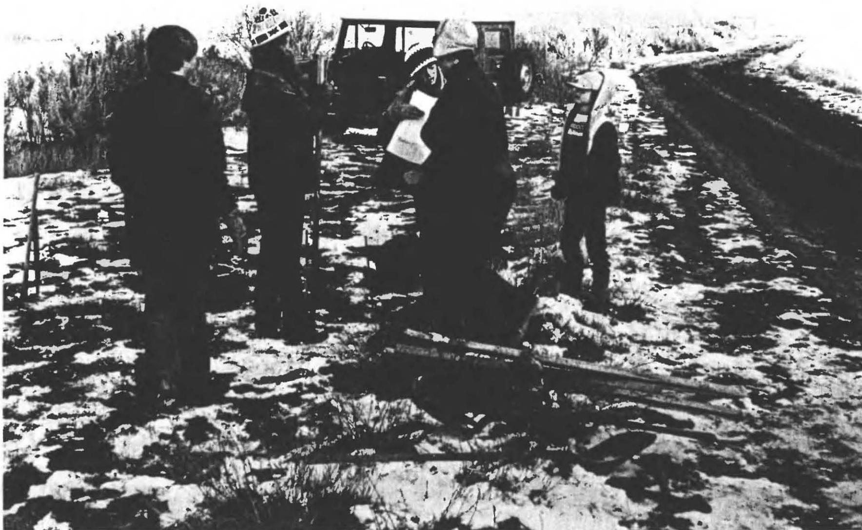
**Fig. 2.2.** Starting to stake out the shelter trench near Montrose, Colorado, at 7:17 AM. The six doors, some tools, water, etc., were carried in a station wagon. The ground was frozen only about an inch deep.
