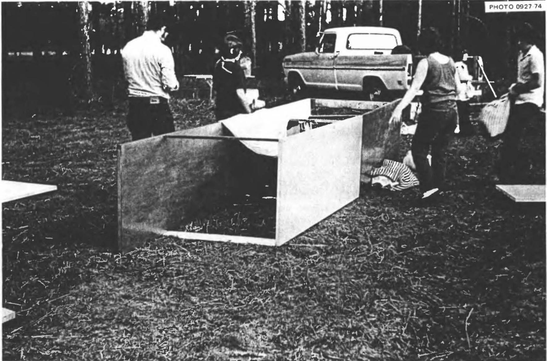
Fig. 5.3. Some of the doors set up as forms around which the earth-filled rolls were built to make the above-ground walls of the 7-person shelter built by this postal clerk, his secretary-wife, their 14- and 12-year-old sons, and their 13- and 9-year-old daughters. Note the cross bracing tacked to the inner edges of the hollow-core doors. These same doors were used for the roof, after the walls made of rolls had been completed.
