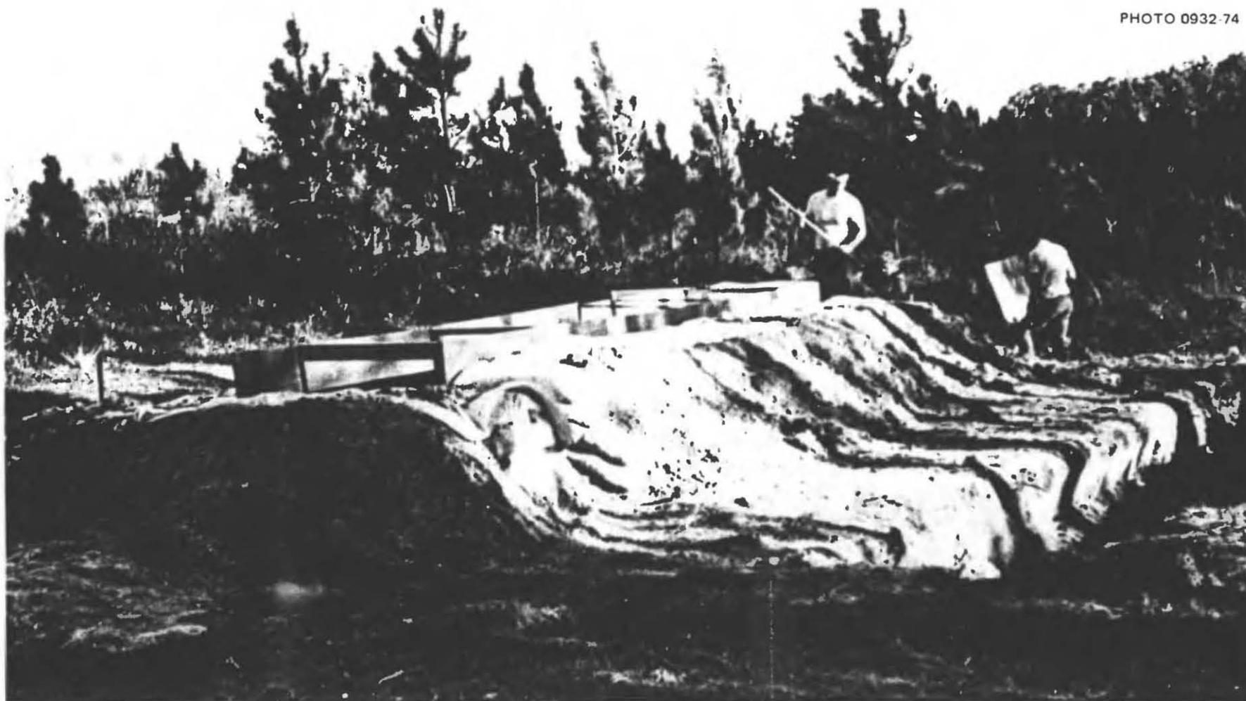
Fig. 5.7. One of the side walls, made of three rolls placed one on top of the other, pictured shortly before the door forms were removed.
