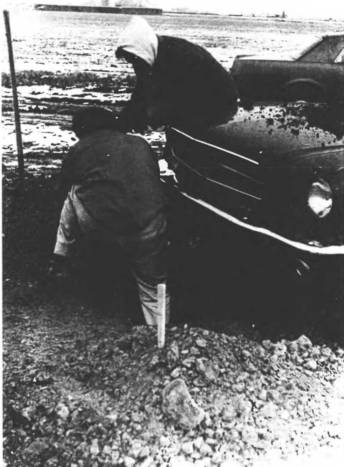
Fig. 6.13. Placing earth-filled plastic garbage bags around the edges of the entryway trench.
