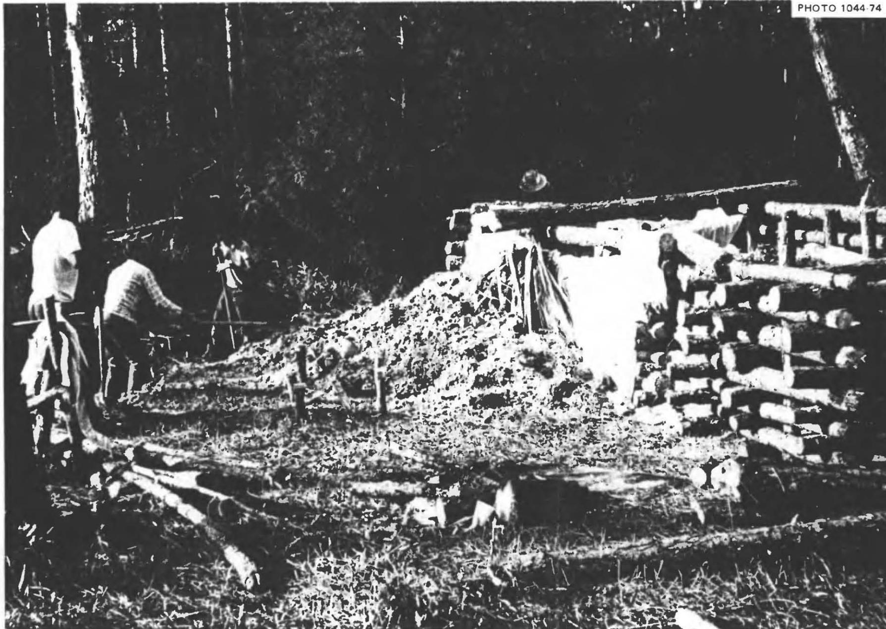
Fig. 5.18. View showing earth being mounded against one of the spaced-pole walls of the shelter. The crib nearest the camera had not yet been lined with a bed sheet, preparatory to filling with earth.
