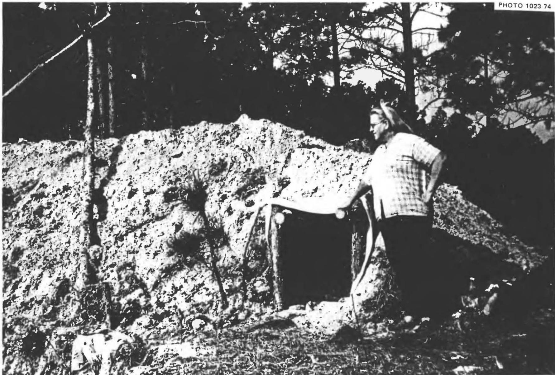
Fig. 5.52. The properly completed entryway of the A-Frame Pole Shelter, pictured on the day following its completion. These hard-working rural families built this 21-person shelter in 12 hours 14 minutes, from the time they received the instructions on a farm about 2 miles from the shelter-building site.
