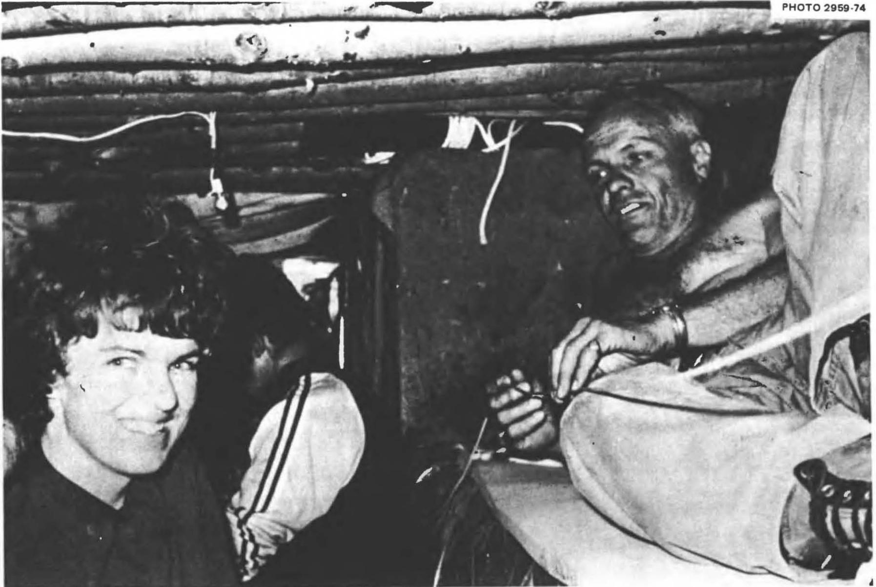
**Fig. 4.14.** Kearny, on his sleeping ledge, pulling the pull cord of the homemade KAP, to demonstrate to Dian Thomas, in the foreground, how a KAP forces an abundant flow of air through a crowded shelter.
