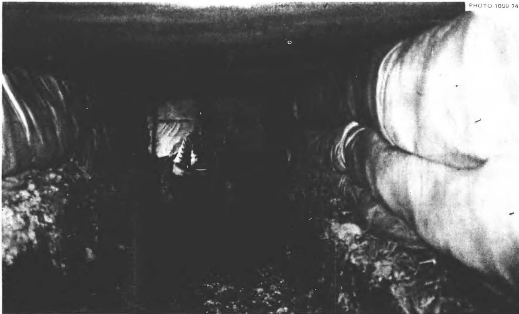
**Fig. 5.12.** Interior of the shelter, showing the roofing doors sloping from the right to the left, and bowed downward about 1 in. due to the 15 in. of wet earth covering them. This bowing occurred as soon as the doors were covered and did not increase during the following days.
