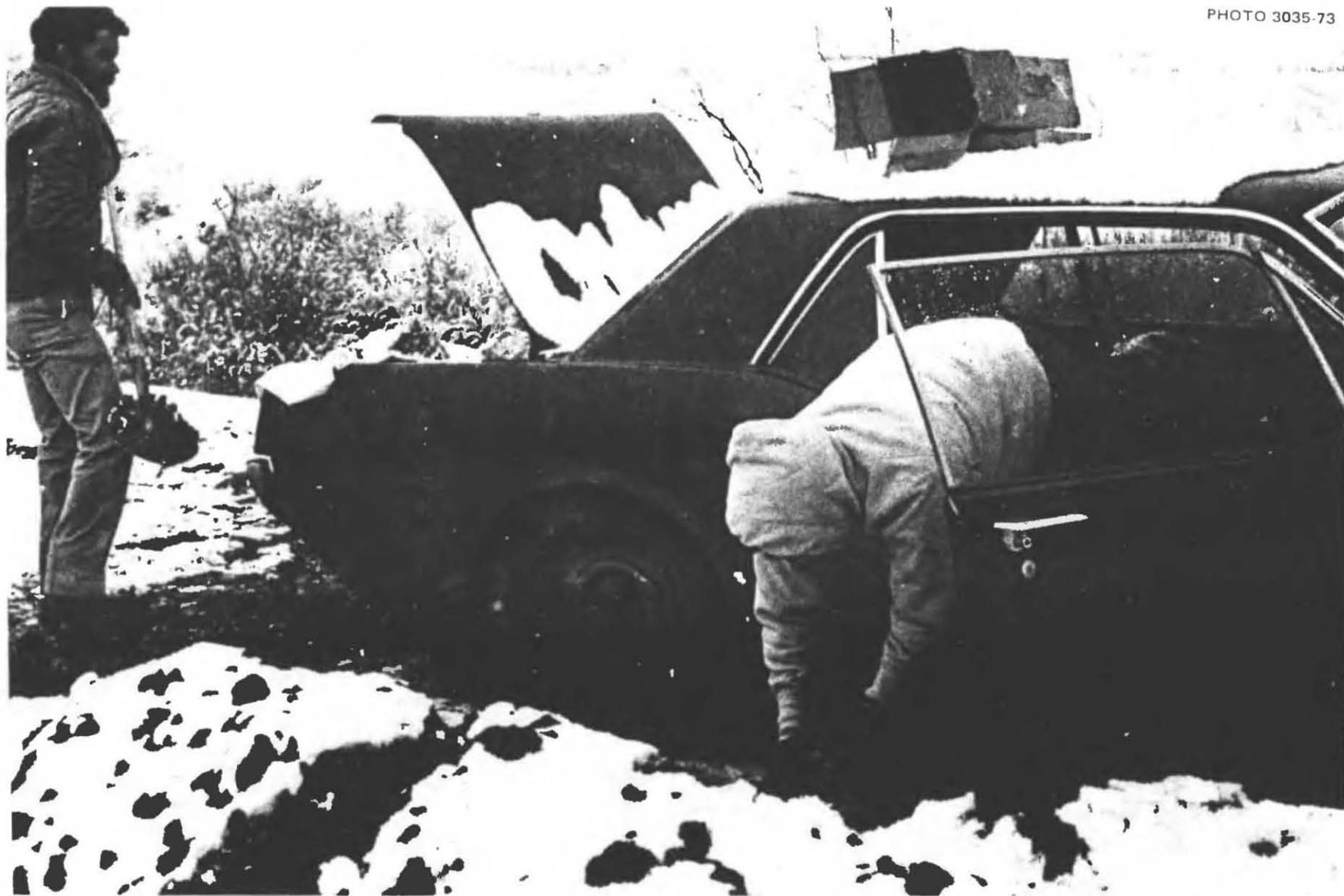
Fig. 6.10. Putting a foot of earth inside the car and in the trunk. Unfortunately, before loading the car with about 2 tons of earth, the father and mother put many of their possessions under their car and on the surface of the ground around the edges of the trench. As a result, when the car body was depressed by its earth load, potatoes in a bag were crushed and cans were pushed into the wet earth near the surface.
