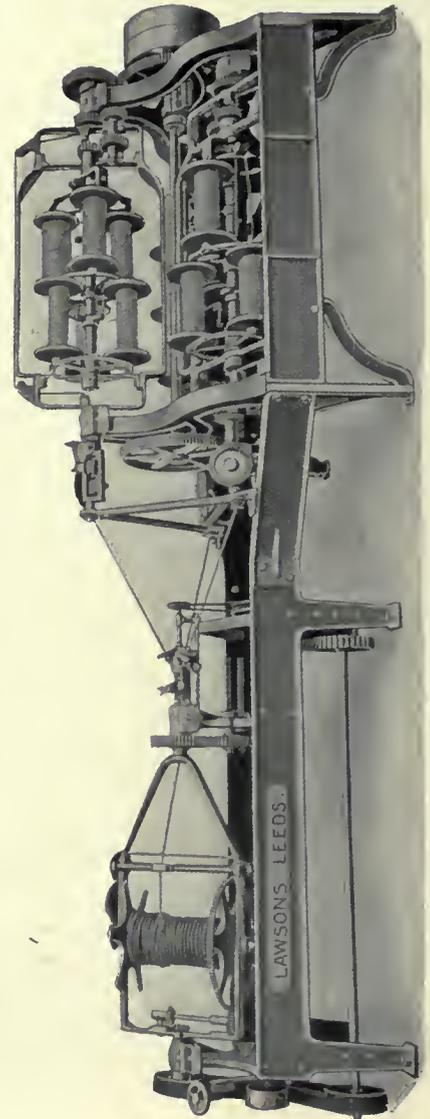
FIG. 17.—EIGHTEEN-THREAD ROPE-MAKING MACHINE.
