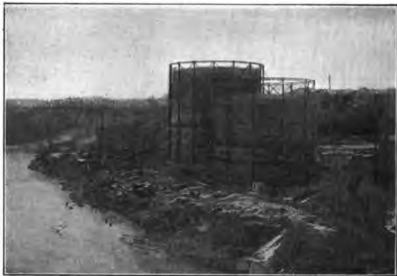
WHY DO WE HAVE GAS TANKS LIKE THIS?
