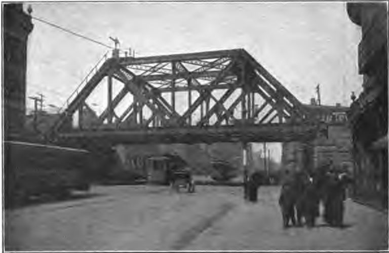
RAILROAD BRIDGE IN NEW YORK CITY
