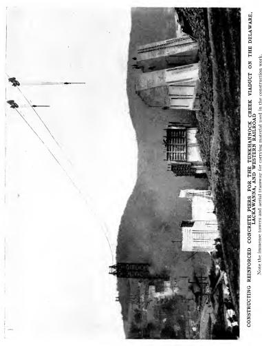
Note the immense towers and aerial tramway for carrying material used in the construction work. Courtesy of Engineering Department, Delaware, Lackawanna, and Western Railroad
