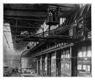
Fig. 109. Wall Jib-Crane, Electrically Operated; Capacity, 10,000 Lbs. Courtesy of Pawling & Harnischfeger, Milwaukee, Wisconsin.
