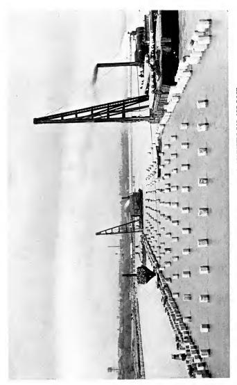
REINFORCED CONCRETE PILES IN PLACE AS SUB-STRUCTURE FOR ORE DOCK A 50-ton test load of pig iron has been mounted on one pile to show whether any appreciable settling resulted. *Contest of Great Lakes Dredar and Dock Company, Chicago*
