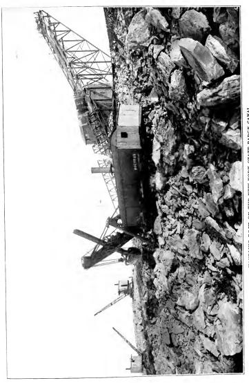
HANDLING ROCK ON THE NEW YORK STATE BARGE CANAL A Bucyrus 70-ton shovel on rock excavator on the line of the canal.
