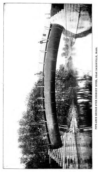
Part of the waterworks system of Boston. Width of span 80 feet, central part of arch riskin 55 feet and bore horizontal. A non-constant and double-rived sections of steel pipe, 5 moh thick and 75, feet in dimeter, sustaining toth its own weight and that of the water it contains. Stone abutment redirected with a backing of the feet of solid/concrete. A larger bridge built on same principle, supported by two arched mains, spans Rook Greek, between Washington and Gorgetown, D. C.
