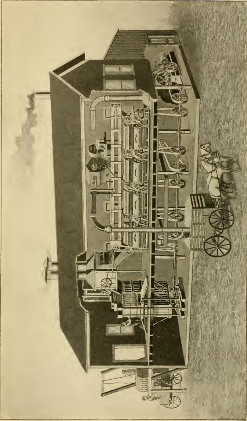
FIG. 26.—Ginnery with Suction Apparatus.
