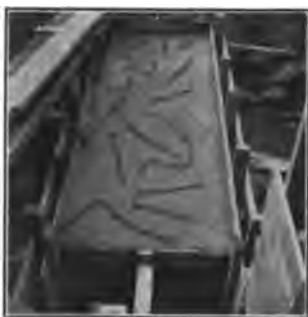
FIG. 5.—Laitance scum at top of foundation slab.
