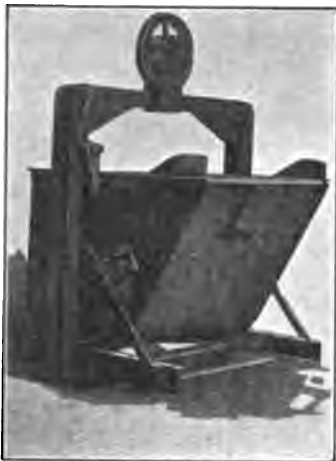
FIG. 32.—Tower-hoist tilting bucket.
