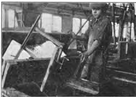
FIG. 113.—Plaster mold with plank pallets clamped on top and bottom being turned over on banker after tamping full, before release of mold parts from the fresh product.
