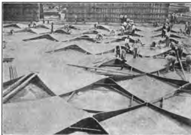
FIG. 51.—Construction view of groined reservoir floor being placed in two layers.
