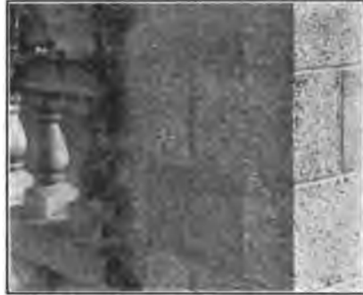
FIG. 118.—Brushed surface. Fine- and coarse-grained surfaces in contrast (crushed limestone).
