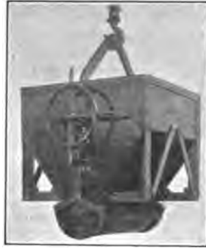
FIG. 31.—Bottom-dump bucket for narrow forms.
