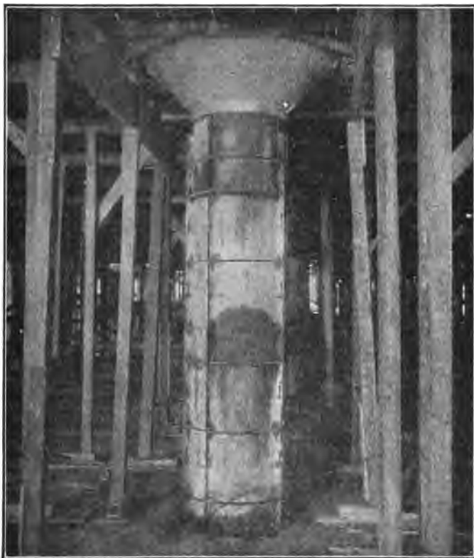
FIG. 53.—Steel column form used in Reid-Murdock Co.'s building, Chicago, Ill.
