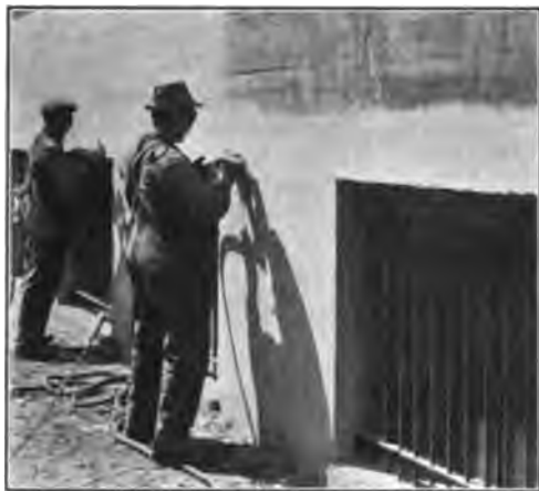
FIG. 21.—Rotary concrete surfacer being used. Note contrast between finished and unfinished surface.
