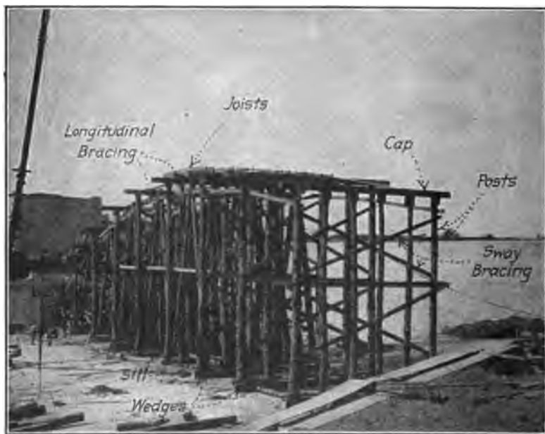
FIG. 41.—Common form of timber centering for arches of low rise.
