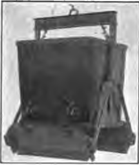
FIG. 30.—Bottom-dump bucket for large forms.
