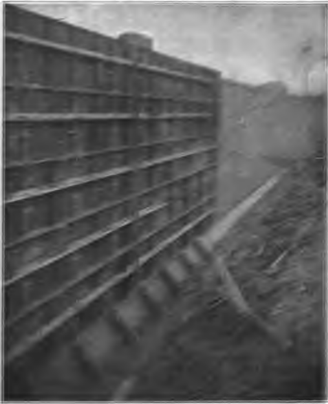
FIG. 71.—Blow light wall forms on foundation wall for plant of Hubbard & Co., Pittsburgh, Pa.
