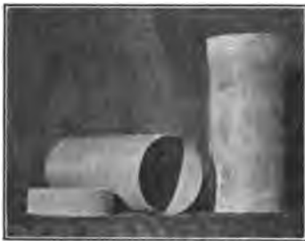
Fig. 8A.—Paraffined paper carton mold.
