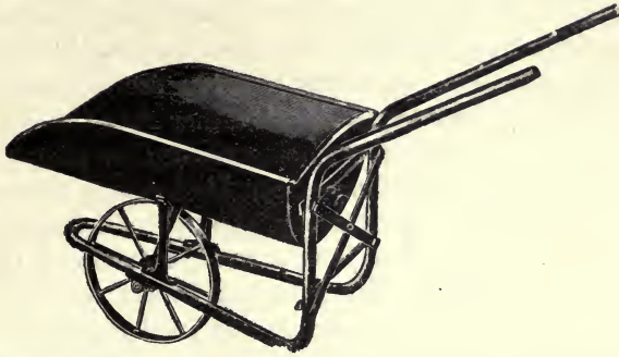
Fig. 16.—Forward Dump Charging Barrow, Sterling Wheelbarrow Co.
