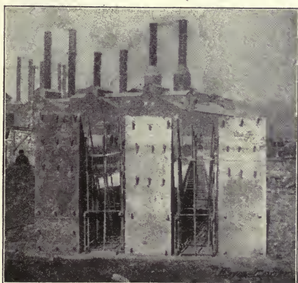
Fig. 240.—Arrangement for Molding Ten Single-Bracket Columns.
