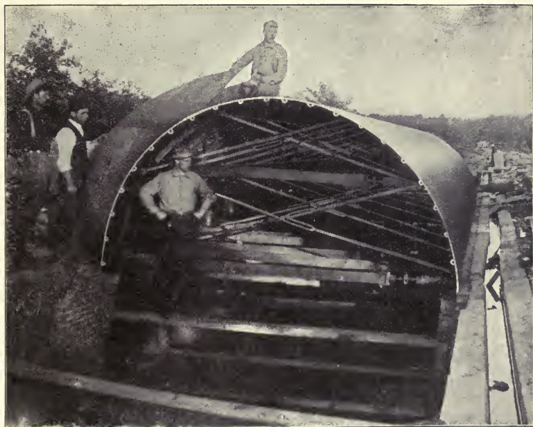
Fig. 247.—Blaw Collapsible Steel Centering for Conduit Construction.
