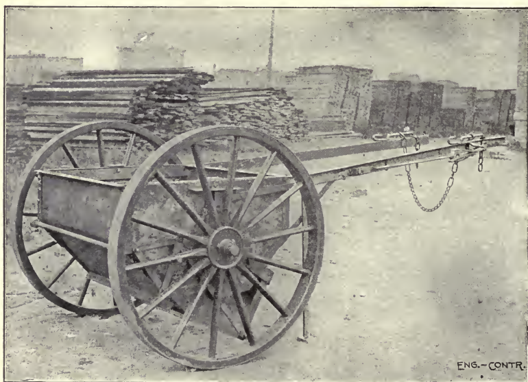
Fig 113.—Briggs Cart Distributing Concrete for Pavement Foundation.
