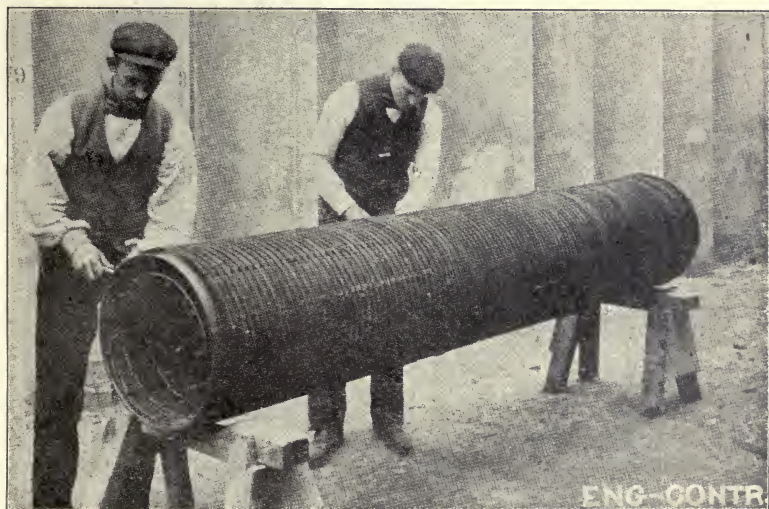
Fig. 271.—Applying External Reinforcement to Bordenave Pipe.
