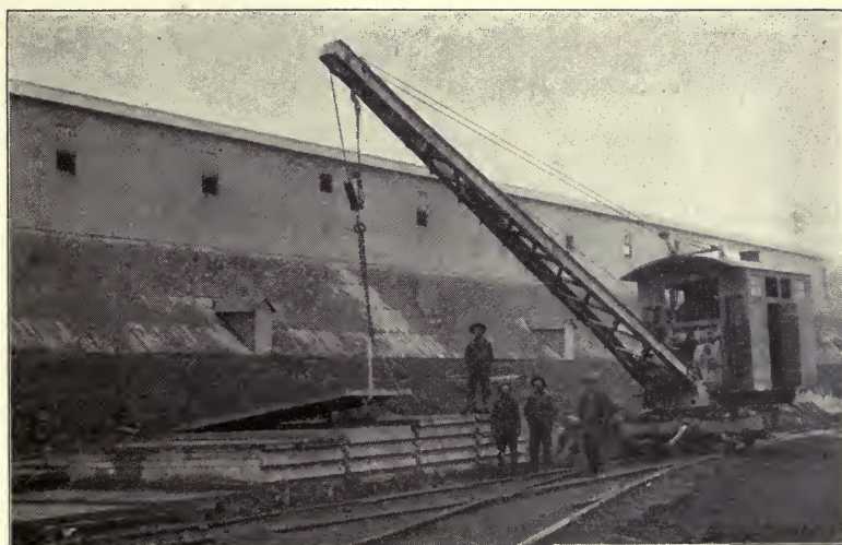
Fig. 245.—View Showing Method of Handling Roof Slabs.
