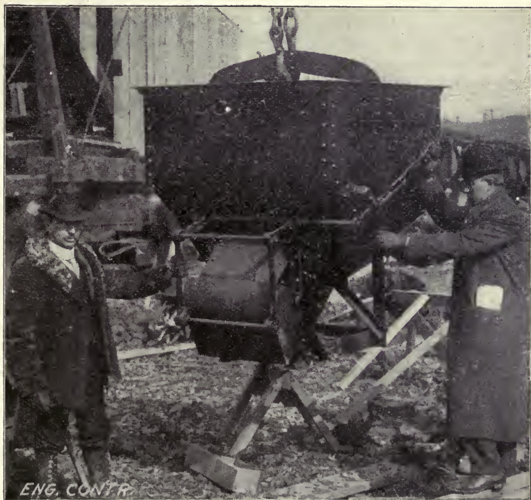
Fig. 222.—Special Concrete Bucket for Large Warehouse Building.
