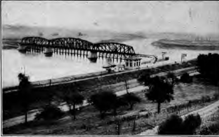
MOVABLE DAM OF THE BRIDGE TYPE AND LOCK
