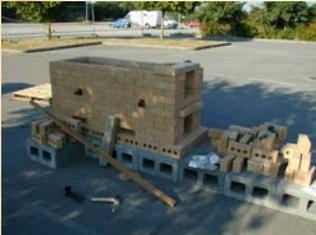
In this picture can see the mouseholes on one side, and the primary air entry at the front.
