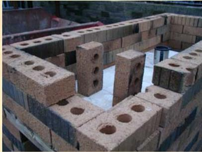
The pot chamber and base of the chimney are now started, and you can see the two support bricks for the chamber side of the chimney. Unless you can use pre fired and shrunk bricks for this, spacers will need to be inserted after the first firing to level things out again, as their shrinkage is considerable. The mug of coffee is not part of the kiln, but it is of course an essential part of the process!
