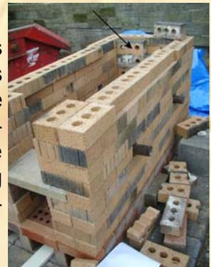
This has now reached the stage where the firebox is complete and the pot chamber and base of the chimney can be built. Notice that the last layer of bricks has been corbelled in to support the base shelves. Notice also the gap at the end of the shelves to allow fire entry from the firebox. In this case it is about nine inches deep and the width of the kiln.
