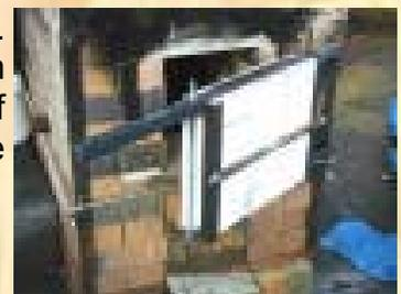
The last thing I do is to make up a mixture of equal parts of scrap clay, sand, and sawdust. Initially this is used to fill up any cracks or unevenness in the joints between the bricks. It can also be used as an insulating layer on the outside of the kiln. You can see some evidence of its use in the last picture on the right. I also use it as a seal between the pot chamber and the thick shelves that make up its lid.
