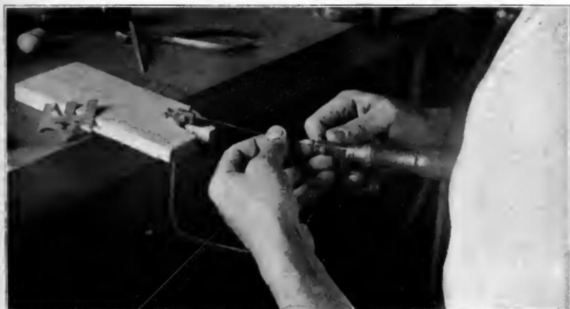
Fig. 29. Placing new blade in saw-frame.
