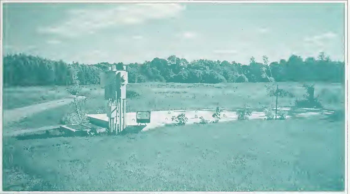
Mechanical plant (RBC)
