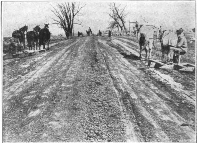
WHEN THE SPLIT-LOG DRAG IS USED AS IT IS BEING USED ON THIS ROAD, THE SURFACE BECOMES RUTLESS AND HARD. NOTE THE STONE DRAGGED TO THE CENTER
