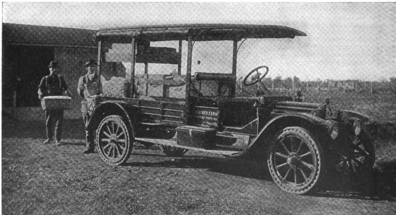
AN IDEAL EQUIPMENT FOR RURAL MOTOR EXPRESS LINES WHERE THE HAUL IS SHORT AND QUICK SERVICE IS DEMANDED. TRUCKS OF THIS SORT CAN MAKE GOOD TIME OVER POOR ROADS AND ARE VERY ECONOMICAL IN OPERATION
