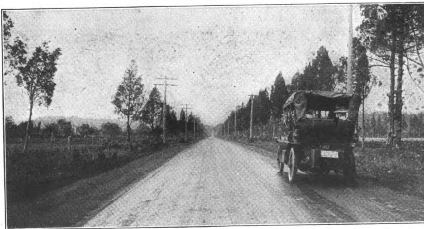
NO MATTER HOW FAST THE AUTOMOBILE GOES IT CANNOT EXTRACT THE BONDING DUST FROM A ROAD LIKE THIS, WHICH IS A PROPERLY BUILT ASPHALTIC, OR BITUMINIZED MACADAM HIGHWAY
