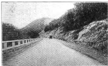
BRICK ROAD COVERED WITH OILED EARTH.
