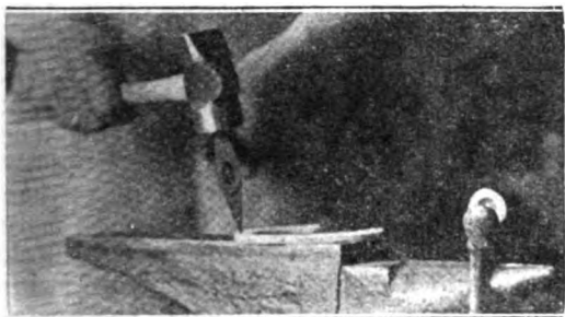
Fig. 14—Punching out nail holes.
