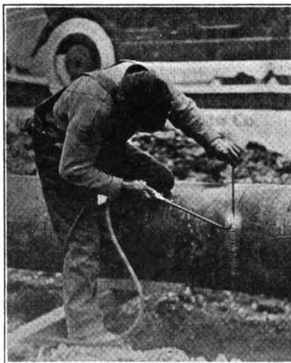
WELDING GAS LINE JOINTS SHOWS BIG ECONOMY. THIS SHOWS A 14-INCH LINE BEING WELDED
