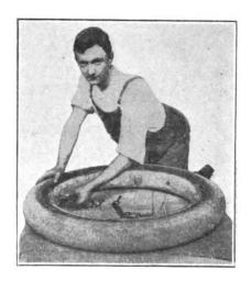
FIG. 5—APPLYING NUTS TO THE SHORT-STEMMED LUGS
