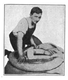
FIG. 2—INSERTING THE TUBE—VALVE STEM FIRST
