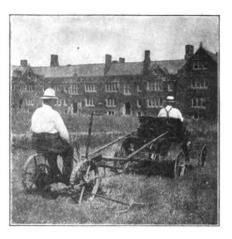
A MOWING MACHINE DRAWN BY AN AUTOMOBILE
