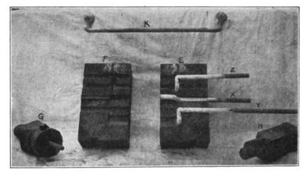
FIG. 7. FREIGHT CAR HAND-HOLDS ARE QUICKLY MADE IN DIES
