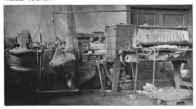
FIG. 5.—SHOWING THE HEATING FURNACE AND THE WELDING MACHINE IN THE WABASH SHOPS AT DECATUR
