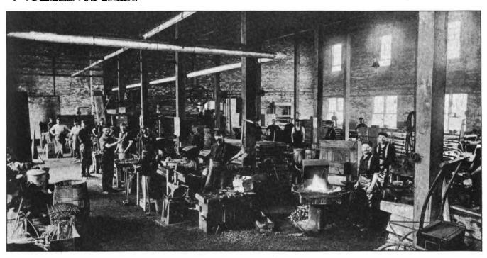
FIG. 9.—THE FORGING, BRAZING, CASE-HARDENING, AND TEMPERING ARE DONE IN THE FORGE SHOP
