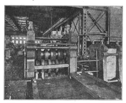
FROM THESE ROLLS THE RAILS PASS TO THE COOLING SHED
