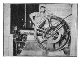
MR. H. B. BERGSTRESSER, OF PENNSYLVANIA, AND HIS POWER PLANT—AN EIGHT-HORSEPOWER GAS ENGINE
