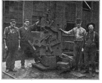
FIG. 3. FOR BENDING WESTINGHOUSE FRICTION DRAFT GEAR YOKES
