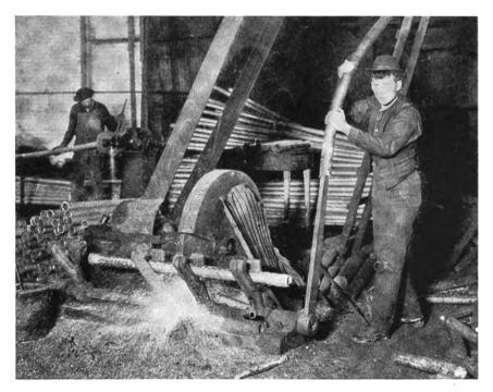
FIG. 4.—SAWING THE PIERCED BILLETS
