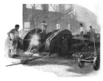
FIG. 1—CENTERING BILLETS BEFORE HEATING FOR PIERCING MILL
