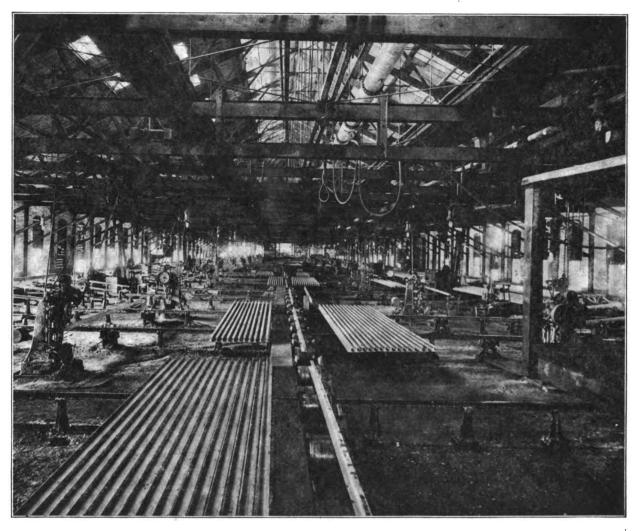
FINISHING SHED SHOWING METHOD OF CONVEYING RAILS
