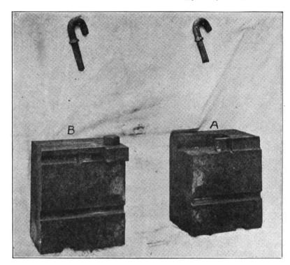
FIG. 9. THESE DIES MAKE THE HOOKS SHOWN ABOVE
