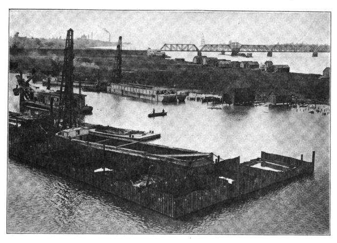
COFFERDAM CONSTRUCTED OF STEEL PLATES MADE BY NEW ROLLING PROCESS
