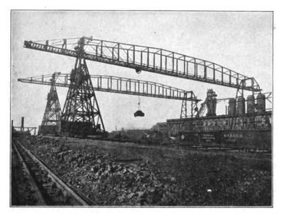
TRAVELING BRIDGE CRANE FOR CONVEYING ORE TO FURNACES
