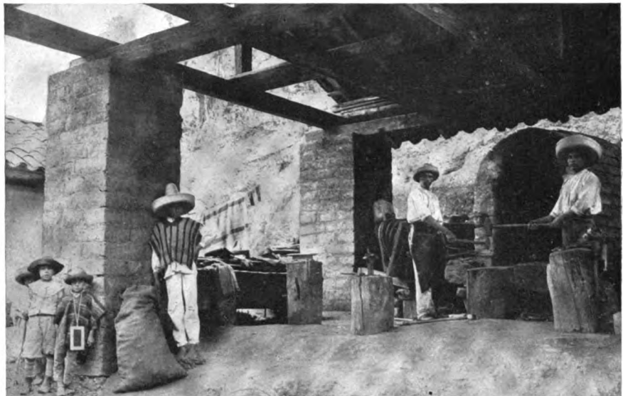
A MODEL MEXICAN SMITH SHOP, WITH ITS ANVILS OF RAILROAD RAIL, ITS PRIMITIVE BELLWOWS, AND ITS VISE FROM "THE STATES"
