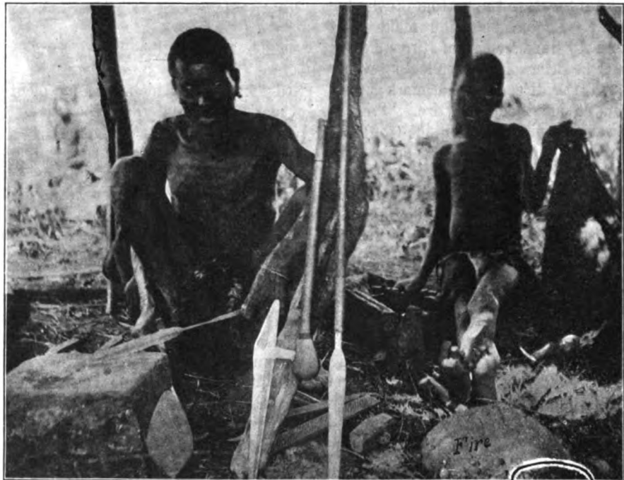
TYANDIRAMBA AND HIS SMITHY, SHOWING FIRE, ANVIL, AND THE WAY HIS HELPER MAKES BLAST.
