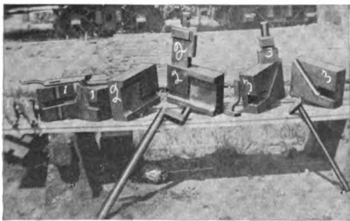
Fig. 2. DIES FOR AN AJAX FORGING MACHINE.
