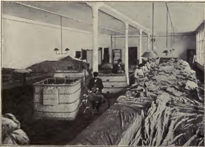
FIG. 108.—Making balloon envelopes in Riedinger's factory, in Augsburg.
