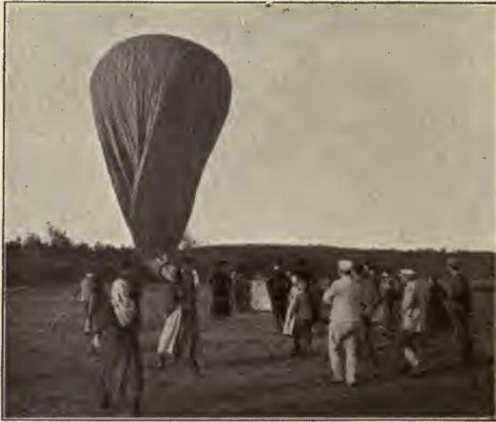
FIG. 126.—Balloon after the ripping-cord has been pulled.
