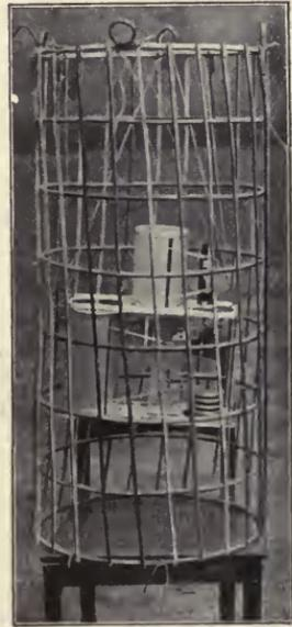
FIG. 158.—A wickerwork basket with instruments for a recording balloon.
