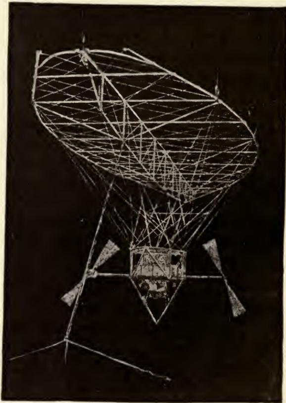
FIG. 40.—Framework and car of Lébaudy's dirigible balloon.
