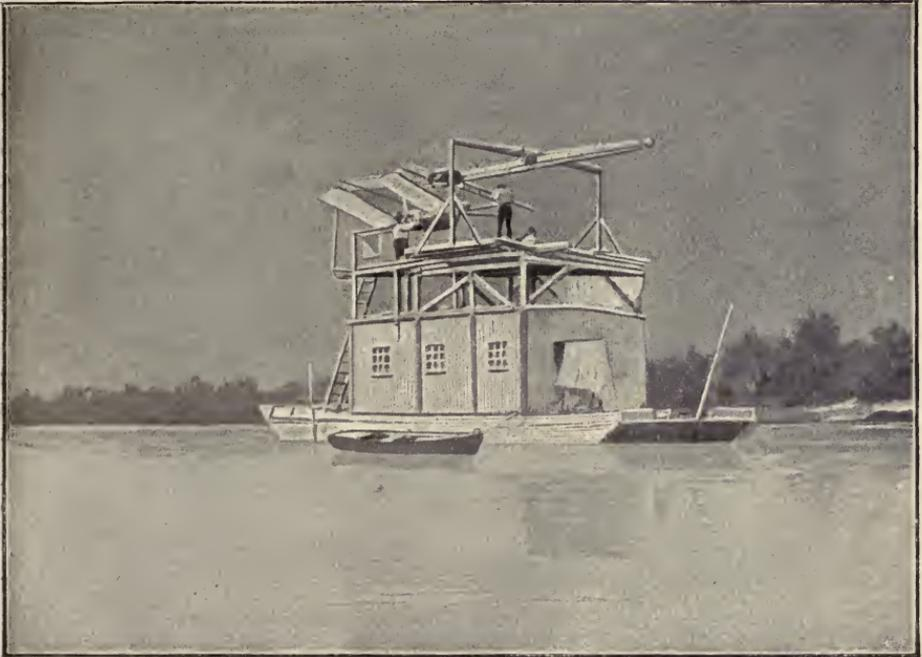
FIG. 56.—Starting arrangements for Professor Langley's flying machine.
