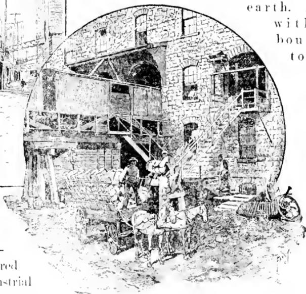
BARREL-HOIST AND TUNNEL THROUGH THE WASHBURN MILL.
