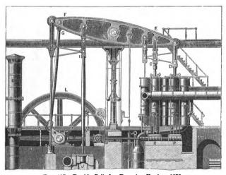
Fig. 105.—Double-Cylinder Pumping-Engine, 1878.
