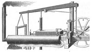
Fig. 46.—Evans's Non-condensing Engine, 1800.
