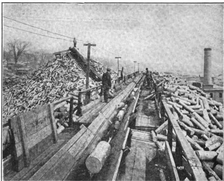
Fig. 21. —Wood storage conveyor showing how sections of trough can be removed and pulp wood discharged from conveyor to accomplish continuous storage.
