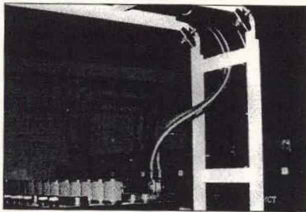
Photo F. A large, well-installed battery bank had the feed cables braced.
