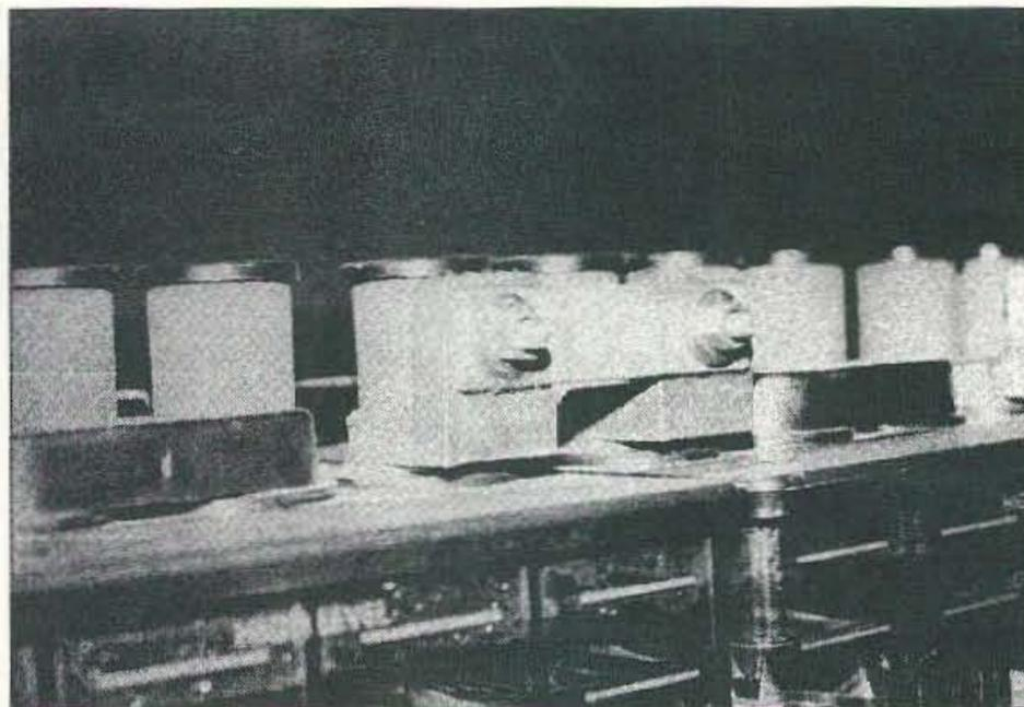
Photo D. These batteries have a flame arrestor vent cap, and access for a thermometer.
