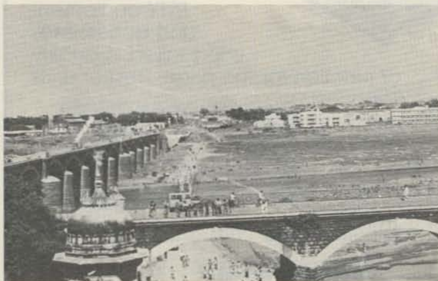
Photo A. The floodplain was swept bare, and part of the bridge destroyed, by the force of the water.
