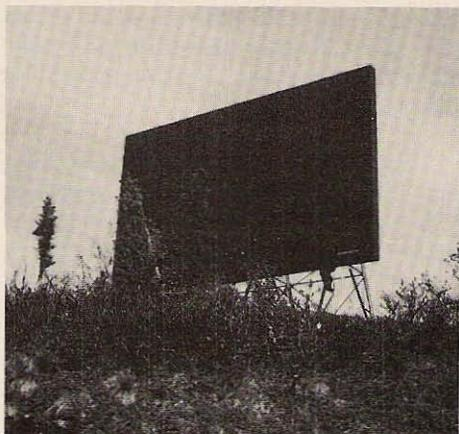
This 30 x 48 passive repeater operates in the 6.7 GHz industrial band, providing service for a commercial microwave system. Installed in Alaska, the passive repeater, with 118.0 dB gain, receives the signal from a station 7 miles away and redirects it to the far station more than 48 miles further on. The system carries 300 voice channels with a measured fade margin of 40 dB.
