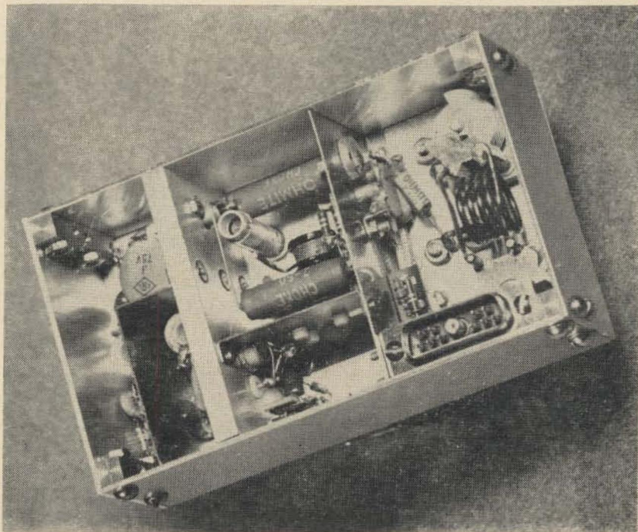
Bottom view of the 48 mc driver. Note Q3 mounted on ¼ inch heat sink/shield with a shield between the base and collector.
