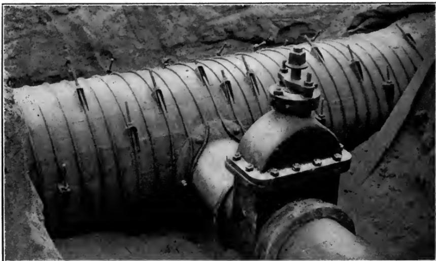
FIG. 30.—Completed redwood stave pipe with gate.
