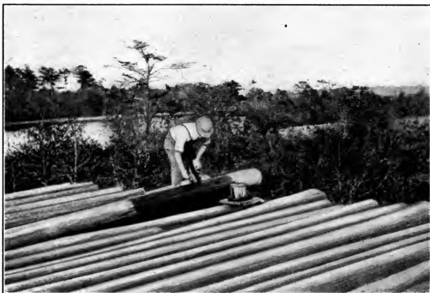
FIG. 75.—Treating poles by brush method.<sup>1</sup>
