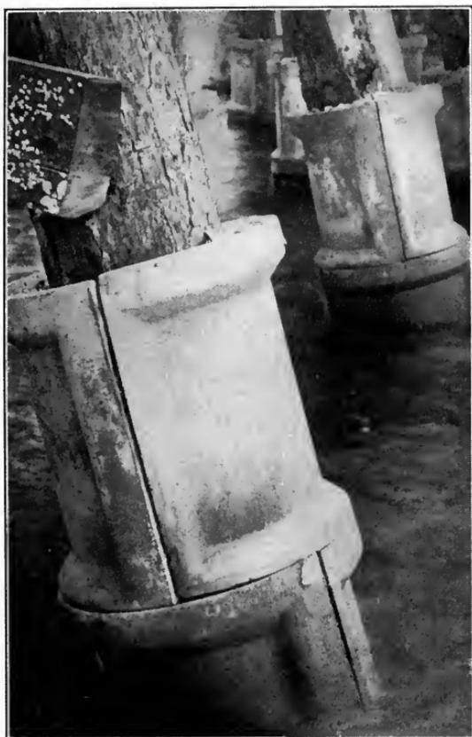
FIG. 61.—Piles protected by pipes and sand.<sup>2</sup>
