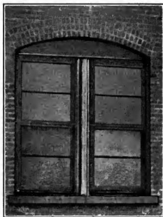
FIG. 48.—Wired glass window in metal sash.<sup>3</sup>
