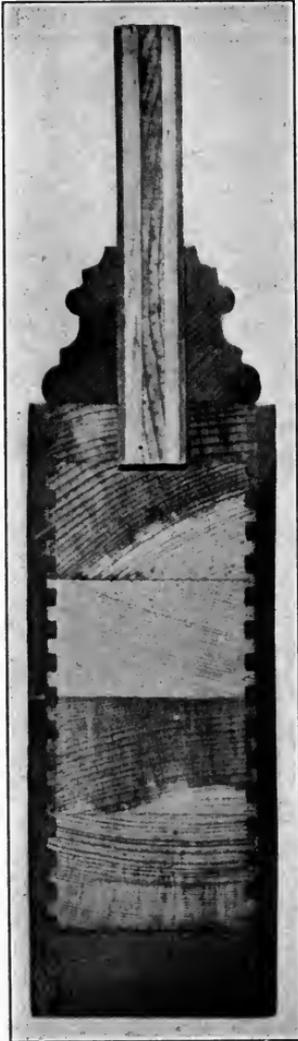
FIG. 84.—Section through door stile.
