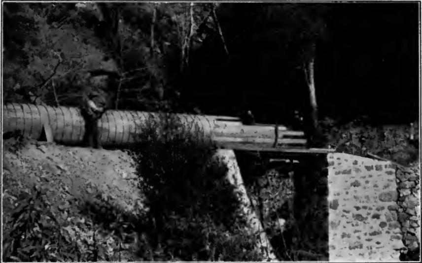
FIG. 29.—Assembling parts of redwood stave pipe.
