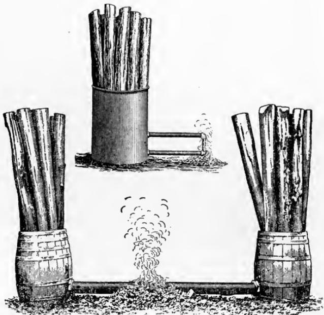
FIG. 77.—Simple apparatus for treating posts.<sup>1</sup>
