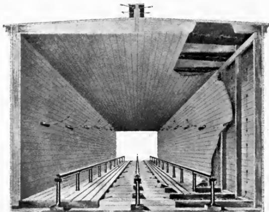
FIG. 69.—Interior of a drying chamber.
