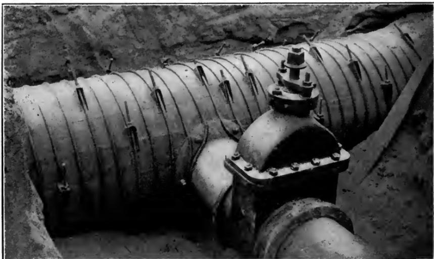
FIG. 30.—Completed redwood stave pipe with gate.
