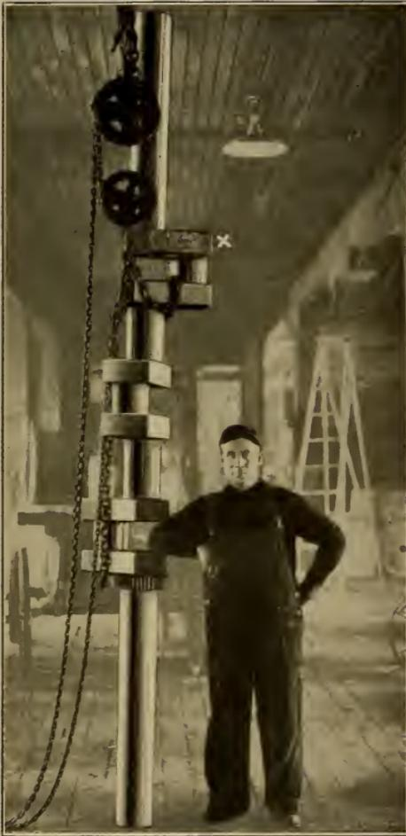
SAME CRANK SHAFT WELDED.
