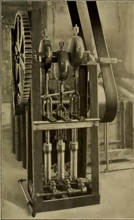
Showing Hydraulic 3 cylinder pump, capacity 12 cub. ft. per minute, compressing oxygen gas from 1500 to 2200 lbs. pressure.
