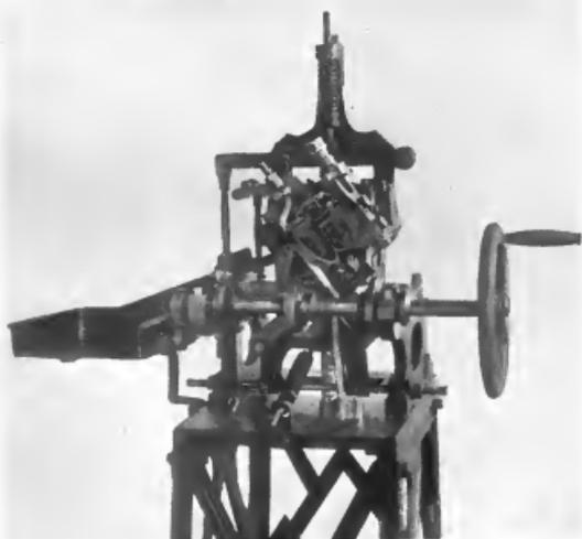
FIG. 288.—Ordinary (English) pivotal typecasting machine. [To face page 302.]
