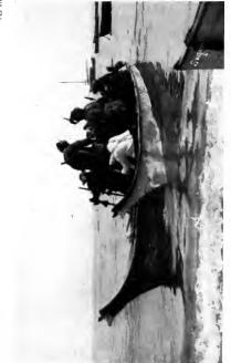
TWO SUQUAMISH "WAR CANOES" LASHED TOGETHER AND CARRYING A PLATFORM OF POLES This device was used in transporting house-planks and for moving large quantities of effects from one site to another. (Photographed at Suquamish, Washington, 1913.)
