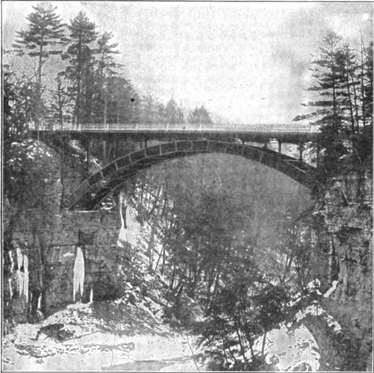
THE FALL CREEK STREET CAR BRIDGE, 170-FOOT SPAN.
