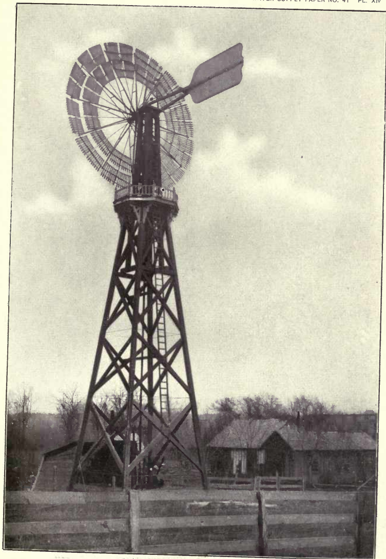
VIEW OF MILL NO. 48—30-FOOT HALLIDAY.
