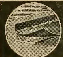
Wall Flashing—Roof Book, page 18, tells how to make it.
