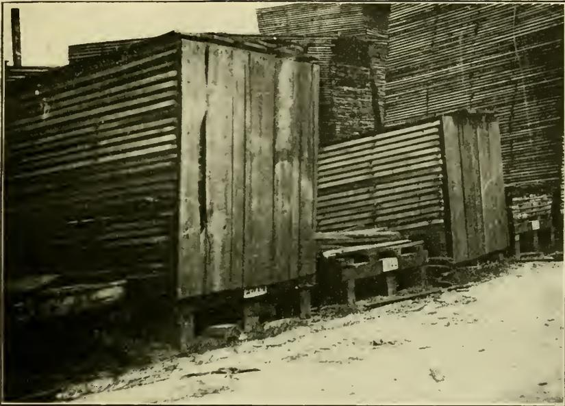
FIG. 1.—SUN SHIELDS USED TO REDUCE CHECKING IN THICK RED OAK TIMBER.
