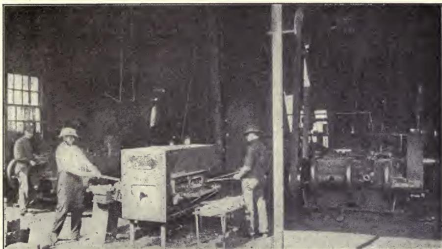
Furnace serving two Bolt Headers. (Note absence of flame from charging openings). A furnace of this type is often placed between a bolt header and a rivet making machine. In either case, it will serve both machines to the limit of the physical endurance of the operators. If desired for rivet heating in larger quantities, various sizes can be heated at one time.
