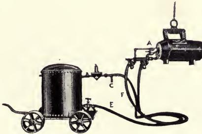
A—Oil burner C—Compressed air connection D—Air reducing valve.
