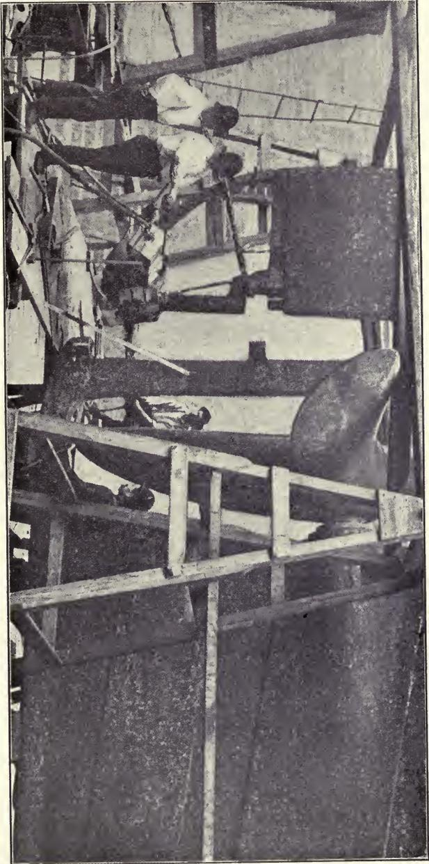
The above is a photograph taken while welding the rudder of the United States Collier "Brutus" while removing the rudder from the vessel. The welding of this rudder was accomplished on August 10, 1905, using the author's equipment.
