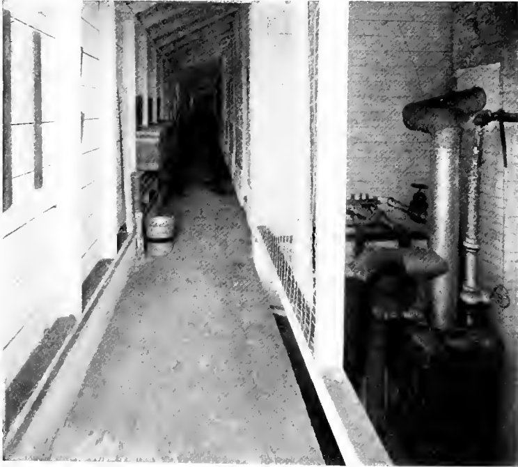
BROODER HOUSE HEATER, WITH WALK AT THE REAR
