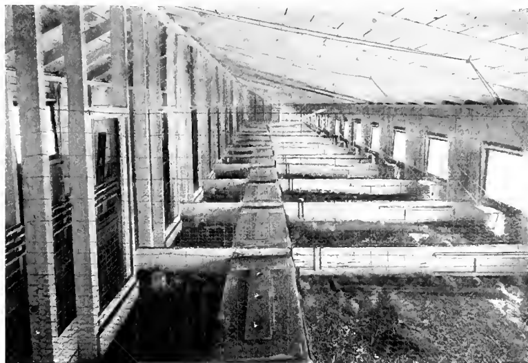
INTERIOR OF HOT-WATER PIPE BROODER HOUSE, SHOWING DETAIL OF PEN PARTITIONS, HOVERS, ETC.
