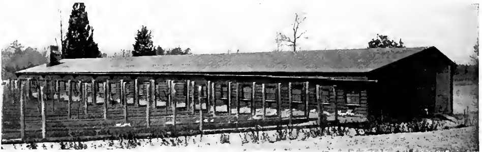
HOT-WATER PIPE BROODER HOUSE, LAKEWOOD POULTRY FARM
