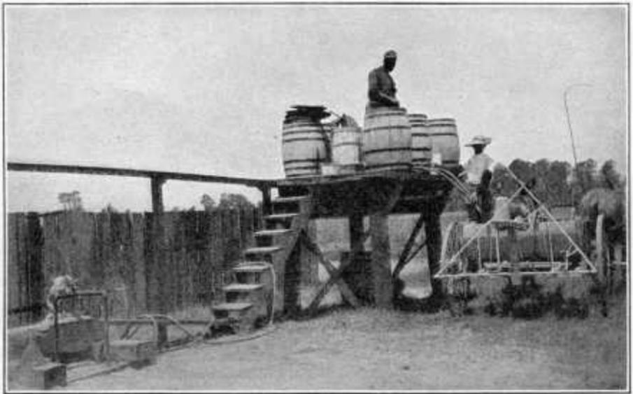
FIG. 6.—An elevated platform, showing a modern arrangement for the preparation of Bordeaux mixture.
