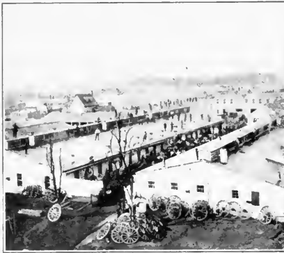
OUTSIDE THE REPAIR SHOPS
