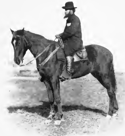
WAUD AT HEADQUARTERS, 1864.
