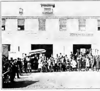
GOVERNMENT TRIMMING SHOP
