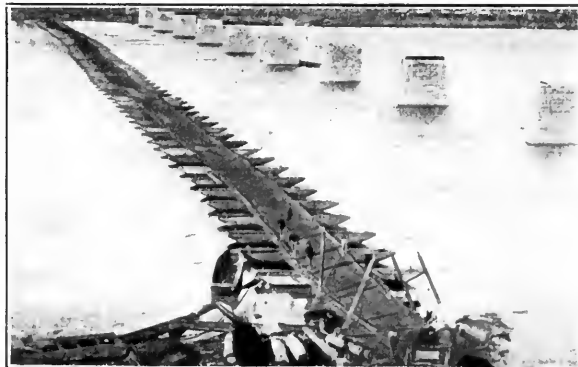
PONTOON-BRIDGE AT DECATUR
