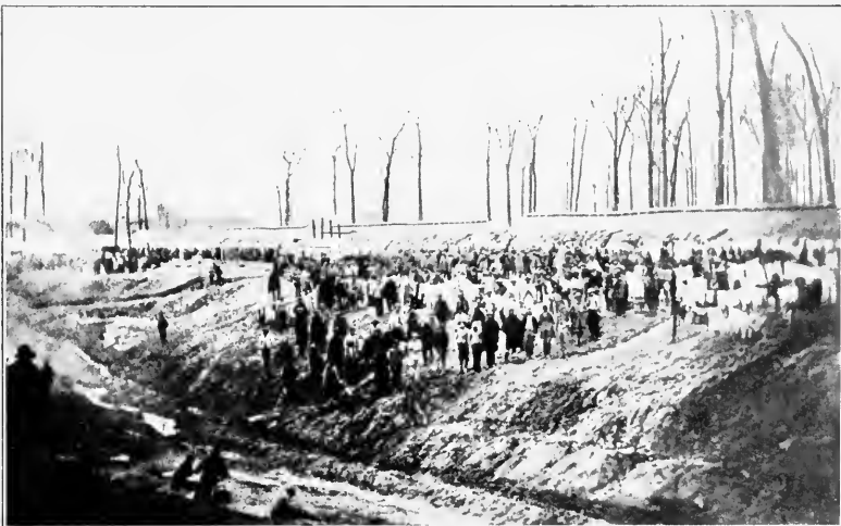
PRIMITIVE DRAINAGE AT CAMP MORTON
