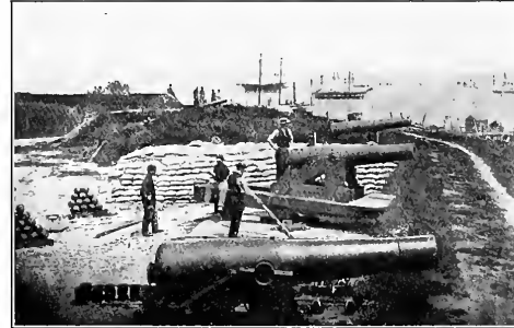
THE CONFEDERATE COMMAND OF THE RIVER. (Battery Magruder, Yorktown.) Looking north up the river, four of the five 8-inch Columbiads composing this section of the battery are visible. The grape-shot and spherical shells, which had been gathered in quantities to prevent the Federal fleet from passing up the river, were abandoned on the hasty retreat of the Confederates, the guns being spiked. The vessels in the river are transport ships, with the exception of the frigate just off shore.
