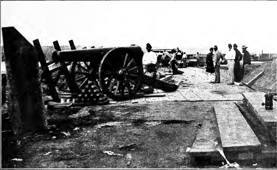
UNCOMPLETED EARTHWORKS, CAMP DEFIANCE
