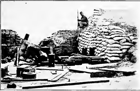
ANOTHER VOICELESS GUN. (Confederate ramparts southeast of Yorktown.) A 32-pounder Navy gun which had been burst, wrecking its embrasure. The Federal soldier seated on the sand-bags is on guard-duty to prevent camp-followers from looting the vacant fort.
