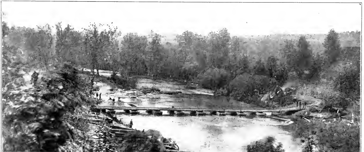
THE BRIDGE FROM UPSTREAM, JERICHO MILLS
