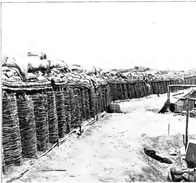
SEDGWICK—GABIONS HEIGHTENED BY SAND-BAGS
