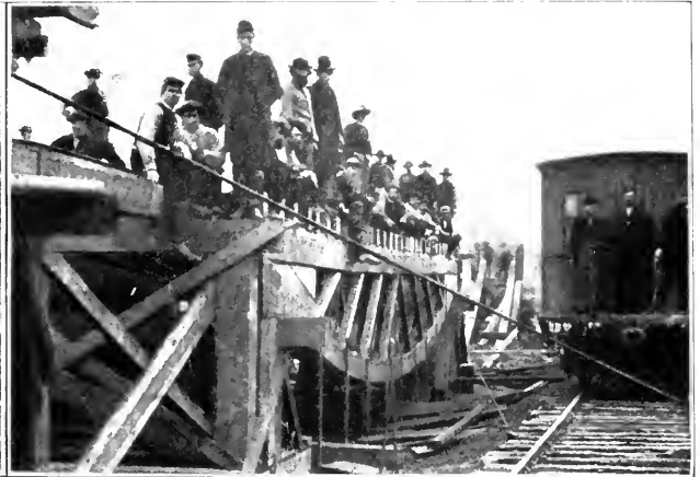
LOADING A BRIDGE TO TEST IT
