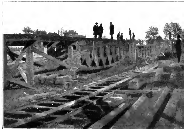
TESTING A "SHAD-BELLY" BRIDGE
