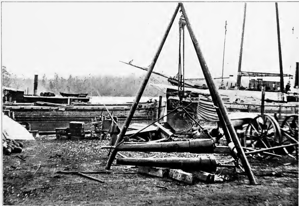
A TRIPOD SWINGING PARROTT GUNS BY THE APPOMATTOX, AT BROADWAY LANDING
