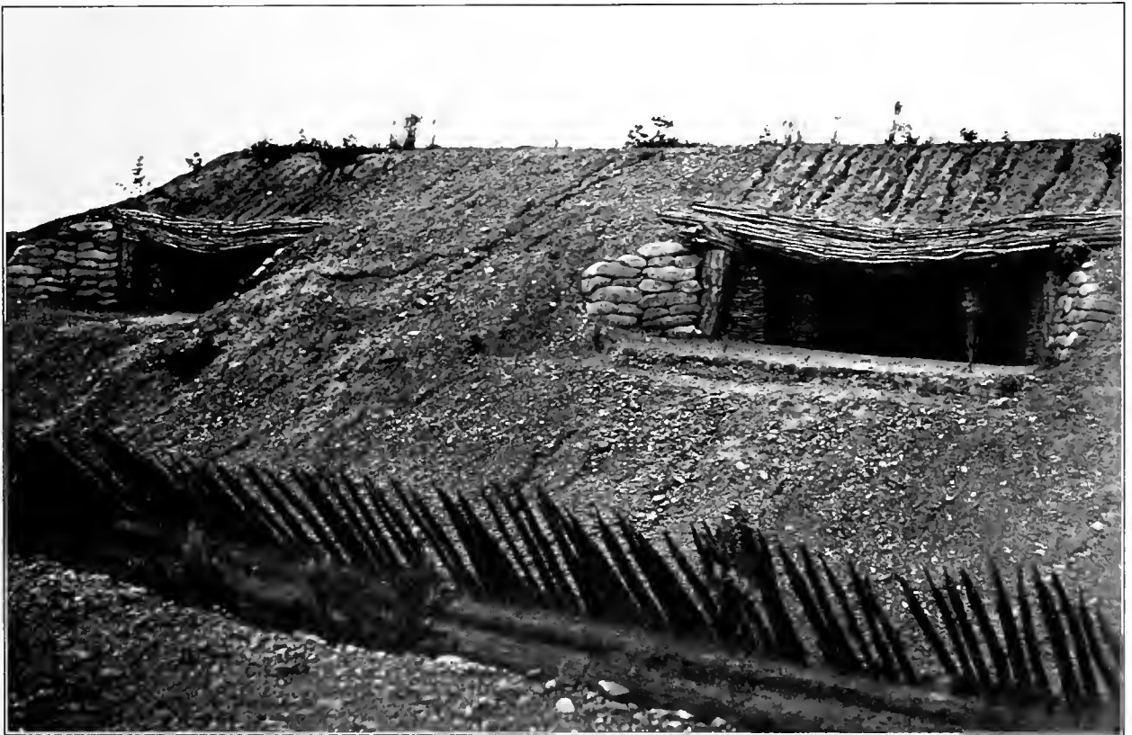
PALISADES AND PARAPET AT FORT HARRISON
