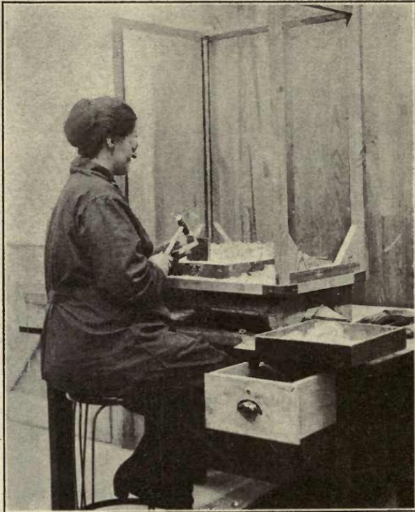
FIG. 52.—Trimming defects from pressed plates of optical glass.
