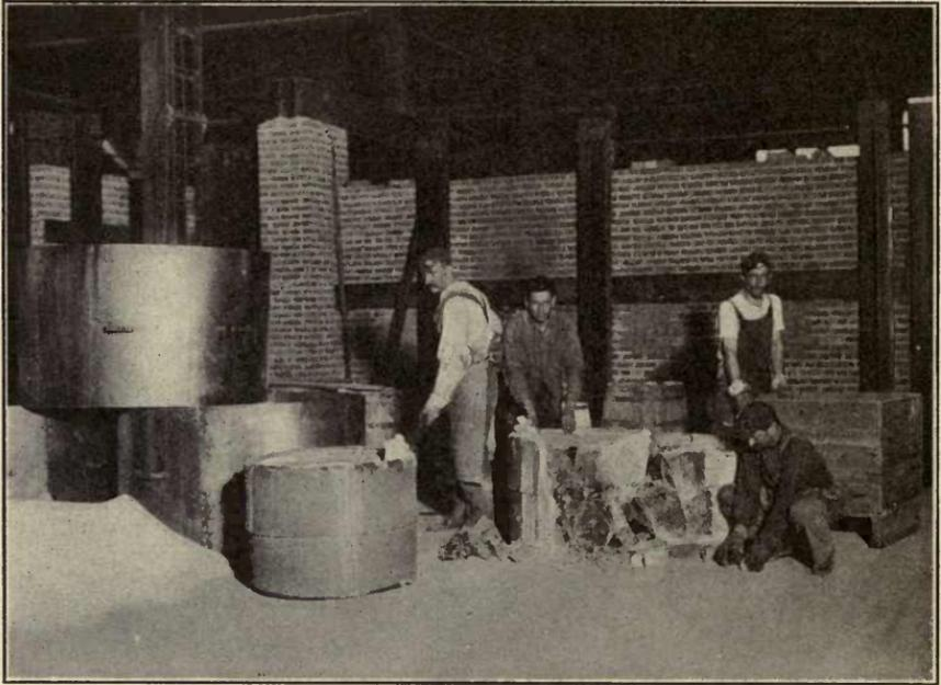
FIG. 48.—Breaking apart pots of optical glass. Note the sheet-iron insulating cap on left, also storage box for pot of optical glass on right of photograph. (Photograph by J. Harper Snapp at plant of Bausch & Lomb Optical Co.)
