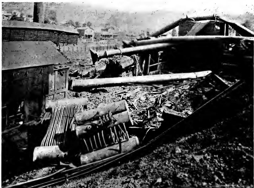
Figure 4—Wreckage at a steel mill following an explosion of a water tube boiler. Caused by external corrosion of one head of the lower drum which had been concealed in brickwork, the explosion killed two people and injured five others. Property loss was about $75,000.
