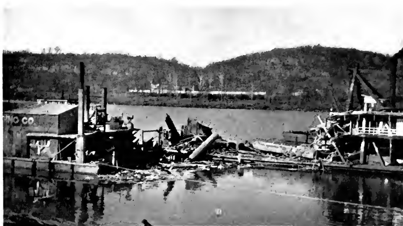
View of the wreckage following a boiler explosion in an Ohio river steamboat.
