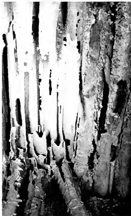
Figure 5—Rear wall of the furnace after forgotten open blow-off valves had drained the tubes.
