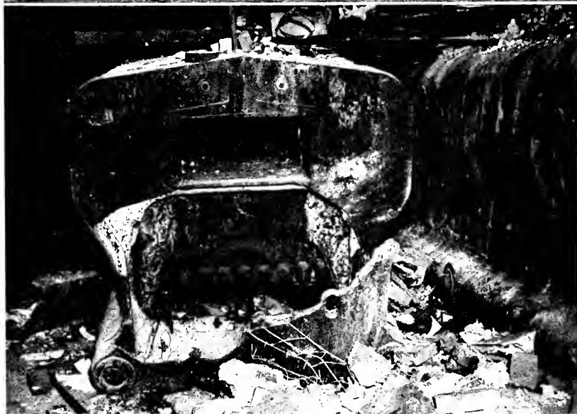
Figure 1—Top—Section of a brick wall in a large apartment house demolished by an explosion in a cast iron steam heating boiler.
