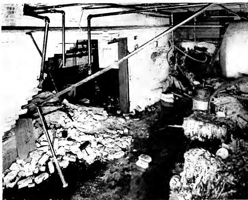
Part of the damage caused by the recent explosion of a condensate receiving tank.
