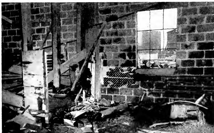
Figure 3—After an explosion of a cast iron hot water heating boiler in a garage. Originally located adjacent to the hole in the rear wall, the base of the boiler was hurled several feet to the right.
