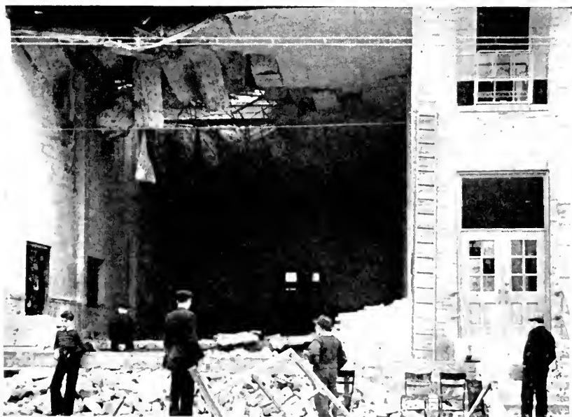
Figure 1—An explosion of a steel hot water heating boiler was responsible for the damage to this Ohio school. Excessive pressure was believed to have been the cause.
