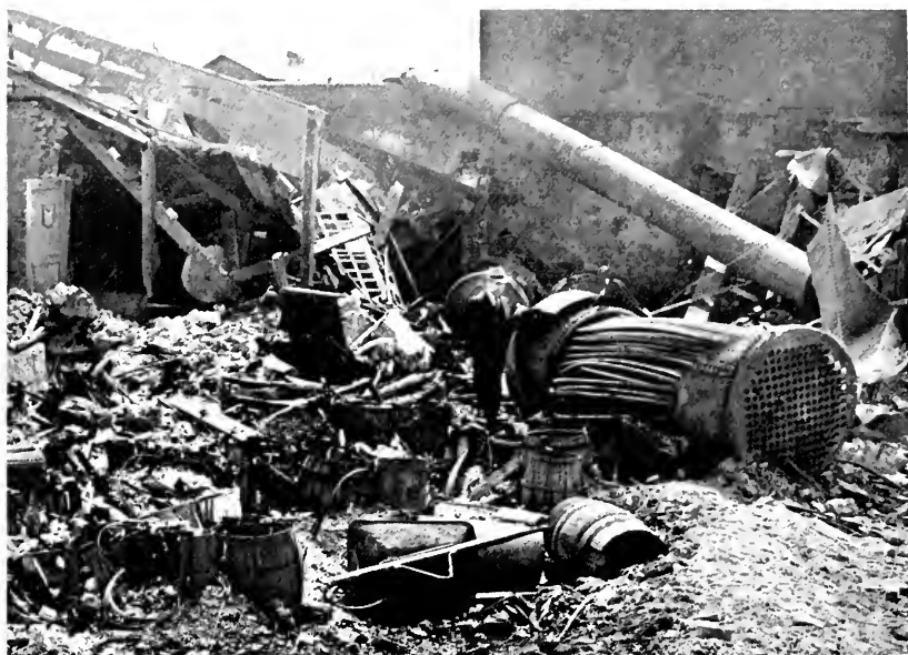
Figure 4—A building demolished by an explosion of a vertical tubular boiler which had been poorly patched by welding.
