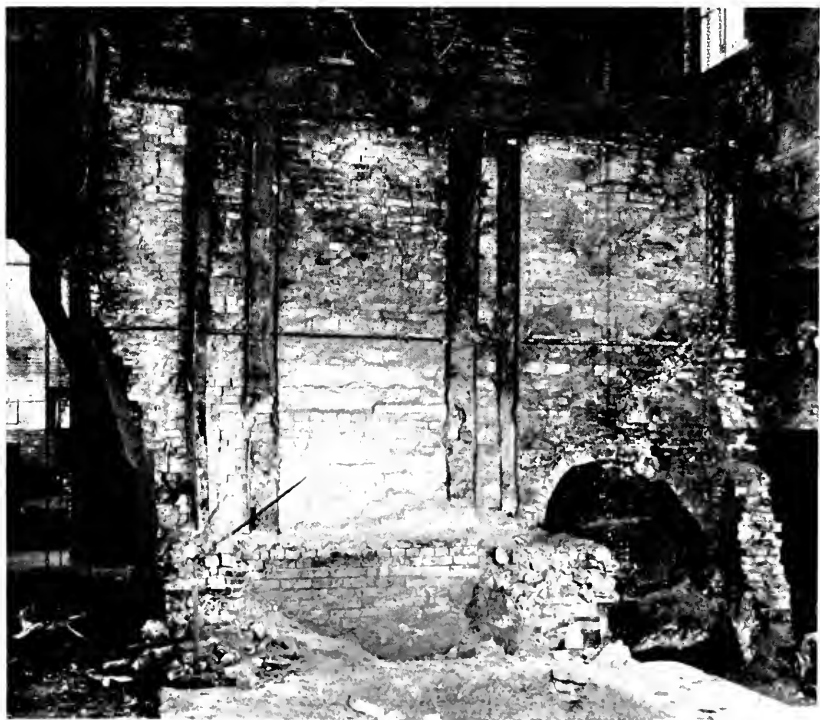
Figure 1—Boiler supporting column, encased in intermediate brickwalls of a battery of boilers, almost entirely wasted away by oxidation from the high temperatures in the combustion chambers.
