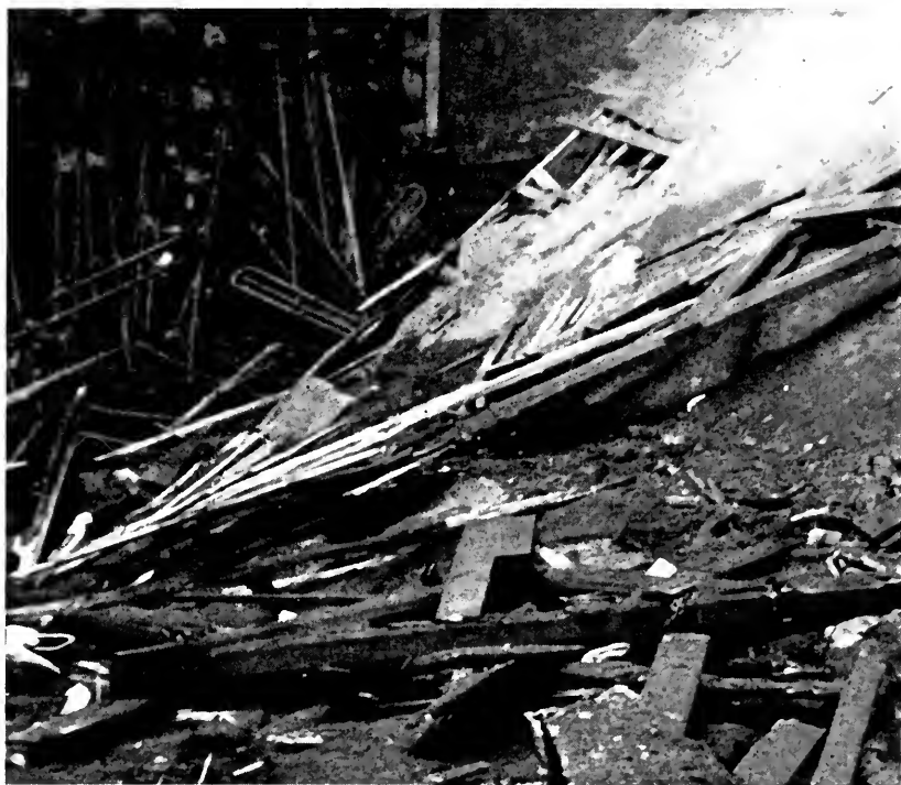
Figure 2—Some of the broken ammonia cooling coils and a section of the collapsed roof following an accident to a refrigerating system in an ice storage building.
