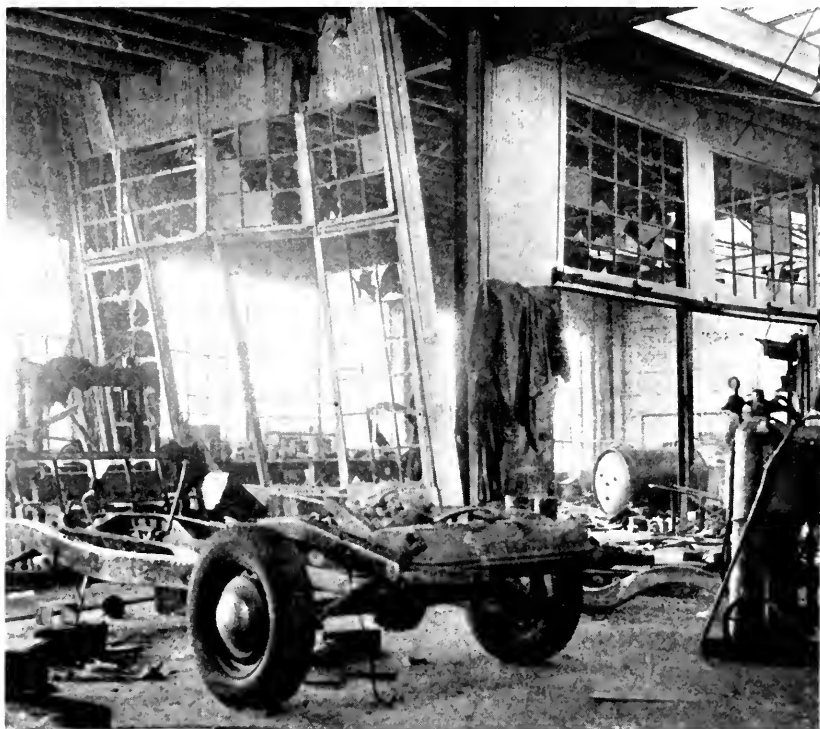
Figure 1—Typical damage as the result of an air tank explosion. This accident occurred in a paint spray room. A workman was injured.
