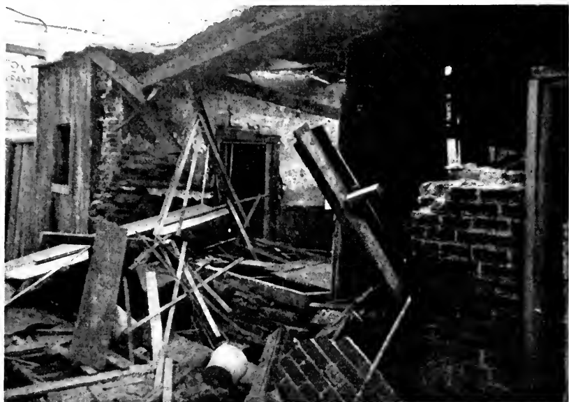
Figure 4—Part of the damage to a laundry building caused by an explosion of a small vertical flueless boiler.
