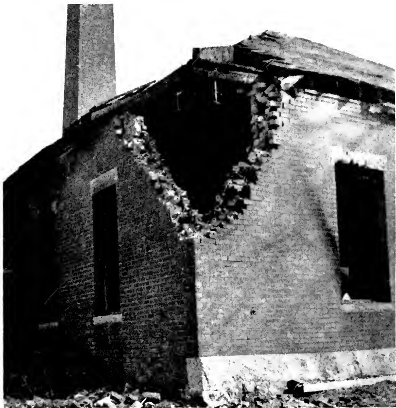
Figure 4—Where an air tank head passed after an explosion. The photograph gives an idea of the force of compressed air suddenly released.
