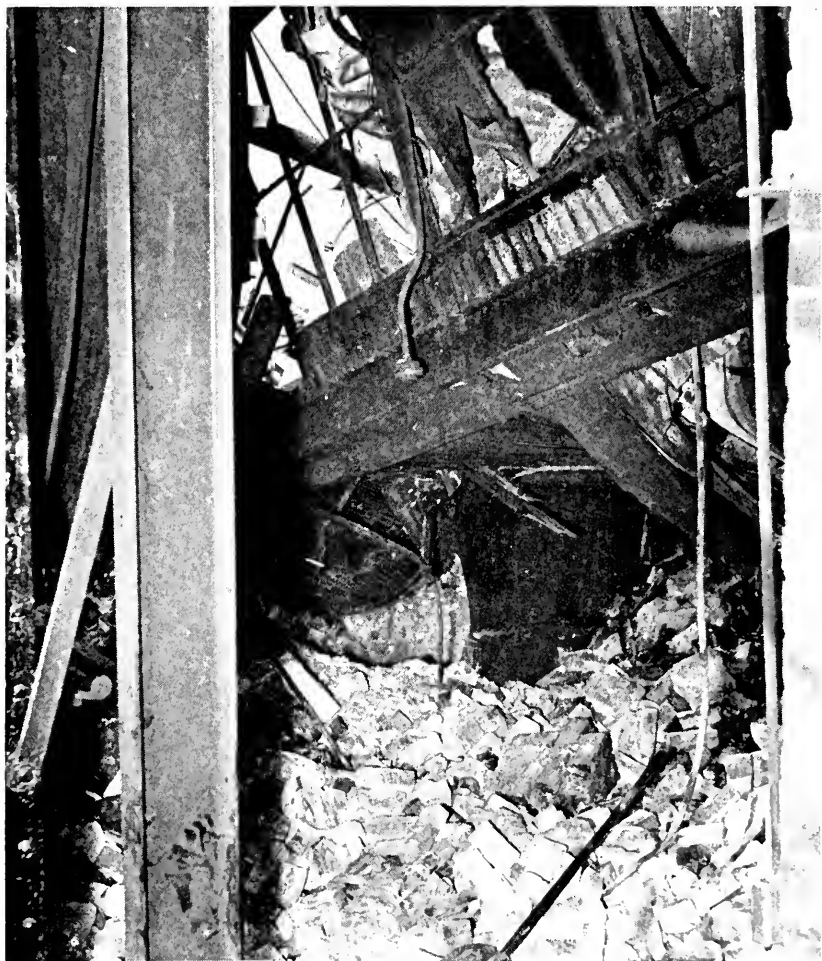
Figure 1—Top page 226—Damage after the explosions of a creosote tank and a water tube boiler at a southern plant.
