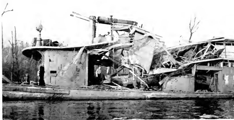
Figure 1—Results of an explosion because of over-heating.
