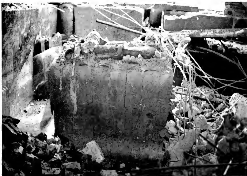
Figure 2—Basement of an automobile showroom after the explosion of hot water equipment. Three automobiles fell through into the basement when the floor was destroyed by the blast.
