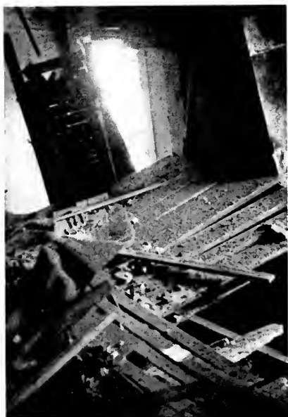
Figure 2—Part of the damage to the first floor of a residence from an explosion of a hot water tank.
