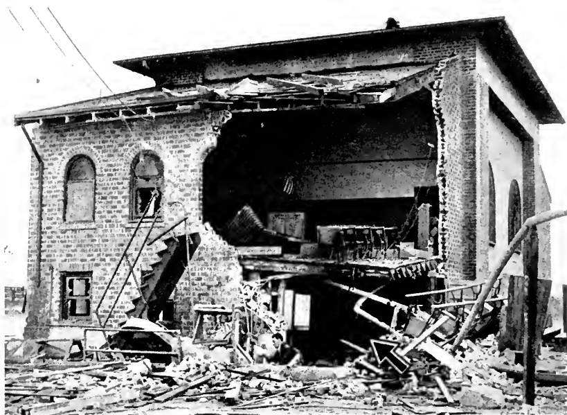
The damage to this school was caused by an explosion of a hot water tank.
