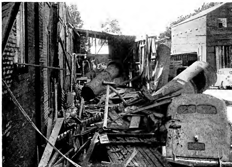
Damage at a creamery and cold storage plant caused by a boiler explosion as a result of low water which, in turn, was attributed to failure of automatic controls. The furnace in the boiler overheated, collapsed and ruptured. Property loss was nearly $5,900.
