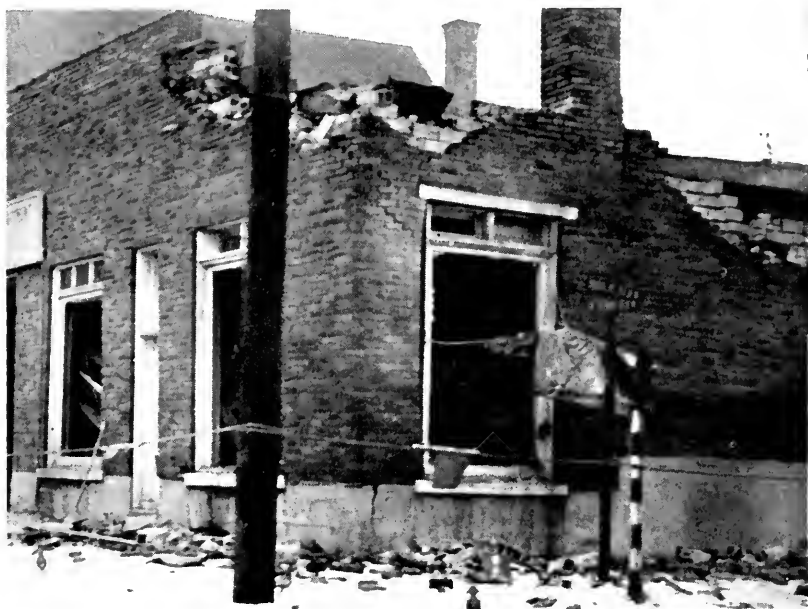
Figure 1—Damage to the exterior of a large garage because of a hot water tank explosion.
