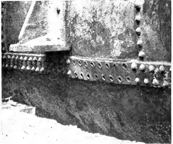
A DEFECTIVE BUTT STRAP DISCOVERED BY INSPECTION.
