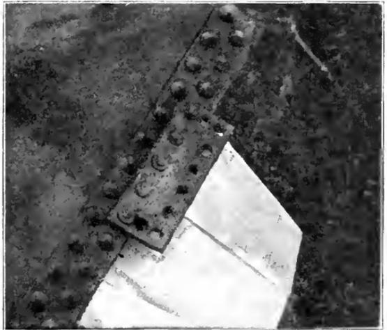
SOFT PATCH USED IN AN UNSUCCESSFUL ATTEMPT TO REPAIR A LONGITUDINAL SEAM CRACK.
