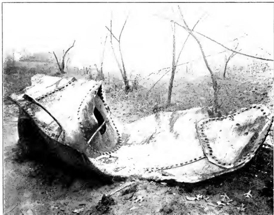
BOILER EXPLOSION CAUSED BY CORROSION.
