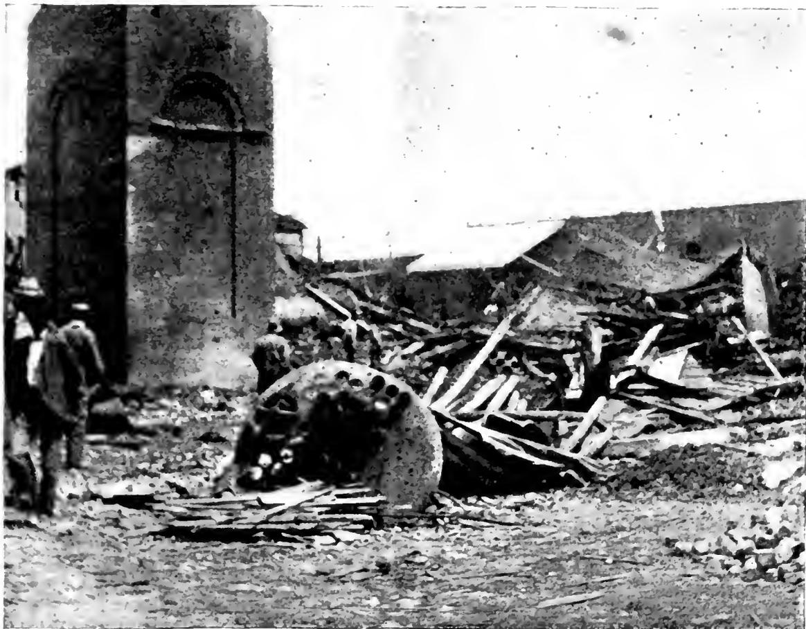
FIG. 3. — SHOWING THE EXPLODED BOILER.
