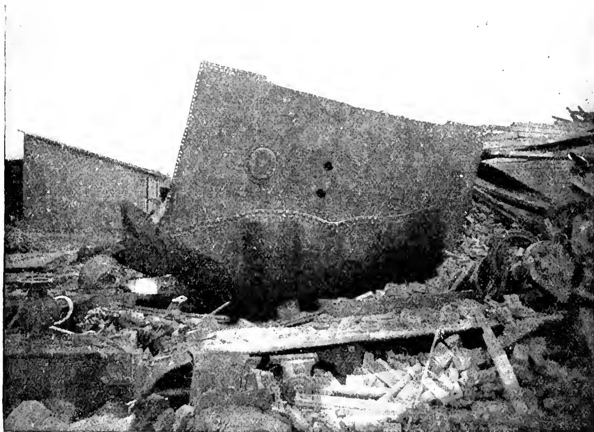
FIG. 2.—SHOWING THE SHELL OF THE BURSTED BOILER.
